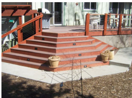
Figure 2. Wide stairs are subject to the same landing requirements as narrow ones.
