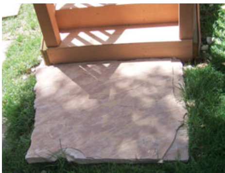
Figure 1. Stair landings must be at least as wide as the stair and at least 3 feet deep. They must provide a safe exit from the stair and may not slope more than \frac{1}{4} inch per foot.
