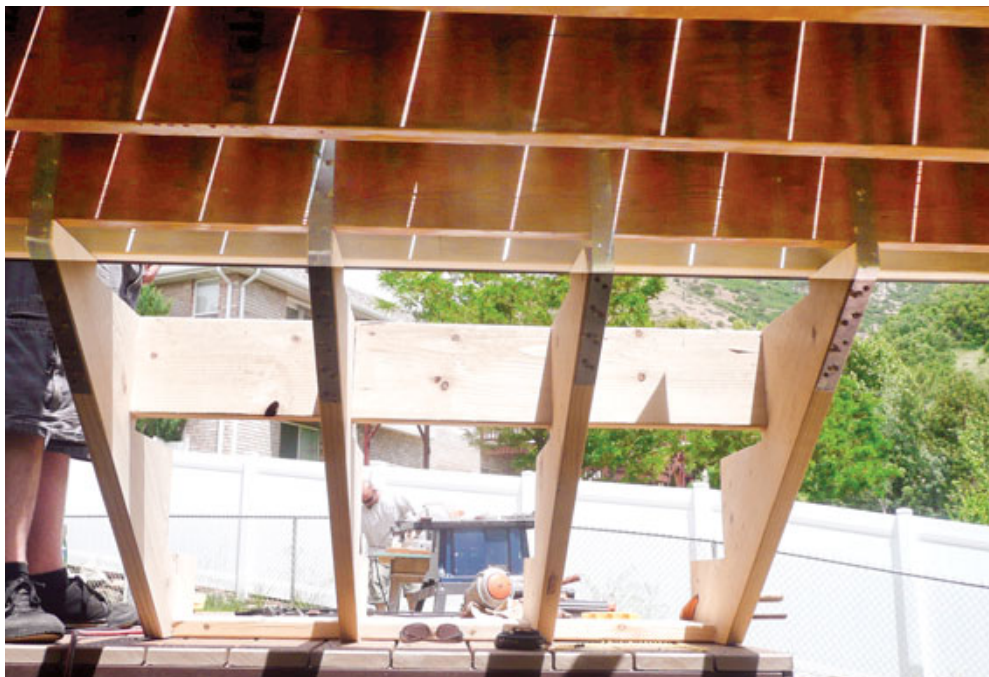
Figure 2. With the jack placed, the strapping is bent upward and nailed to the side of the joist. Use full diameter 10d x 1½-inch nails for the joist connections.
