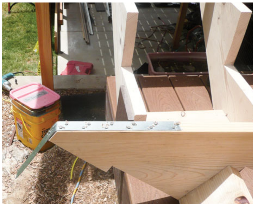
Figure 1. The stair jack, or stringer (foreground, upside down), is cut to extend below the joists. Galvanized-steel strapping is nailed to the jack's bottom with 10d commons.
