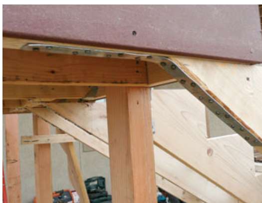
Figure 3. When joists are parallel to the jacks, install blocking between the joists to receive the strapping. The strapping is nailed to the bottom of the outer joist with 16d commons; the combined strength of the inner connections compensates for this somewhat sketchy one.
