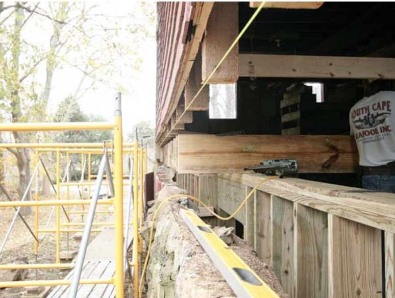
Figure 5. According to the permit, the historic stone foundation at the rear of the barn had to be preserved. Rather than rebuild it, the crew opted to cantilever the new floor framing (top left) over a pressure-treated pony wall set on a reinforced footing poured just inside the stonework (top right). A string line provided orientation for the joist ends, set back 3 inches for a double rim joist (left). With mortar closing the gap, the addition appears to bear on its original foundation (above).
