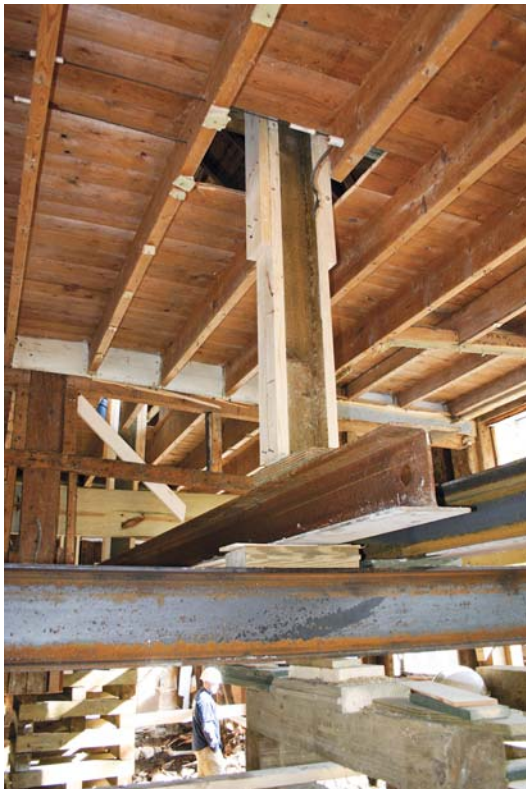
Figure 3. Built-up posts ran from a pair of 20-foot I-beams through the second-floor framing (above) to the roof purlins (above right). This arrangement allowed the roof framing to be jacked independently of the walls. Three-ton chain hoists stretched between the top plates helped pull the walls back toward plumb as the sagging roof was lifted (right).
