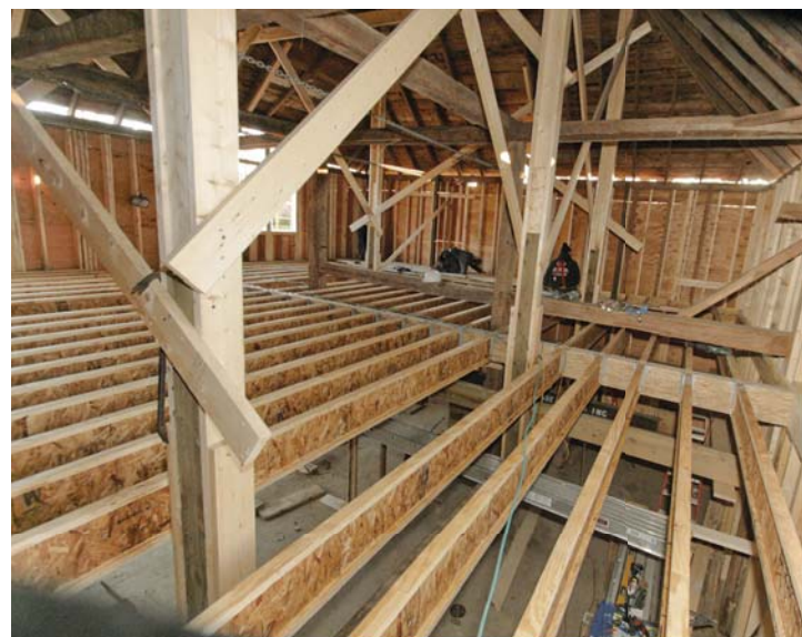
Figure 6. The new first-floor framing had to be installed around the cribbing (left). To fill in the gaps, the crew repositioned the cribbing above and below a completed floor section, then transferred the beam loads to the new stack (below left). With the first floor and wall framing replaced, only the roof supports remained to shore the structure while the second-floor joists were installed (below).
