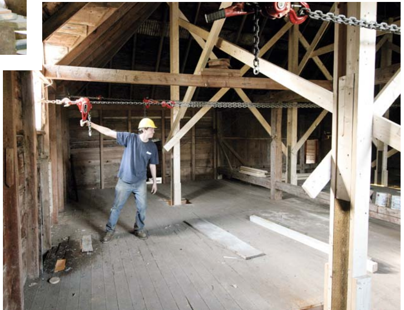
Figure 3. Built-up posts ran from a pair of 20-foot I-beams through the second-floor framing (above) to the roof purlins (above right). This arrangement allowed the roof framing to be jacked independently of the walls. Three-ton chain hoists stretched between the top plates helped pull the walls back toward plumb as the sagging roof was lifted (right).
