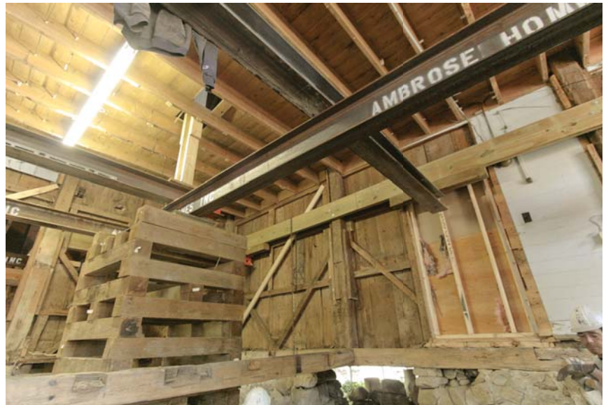
Figure 2. The eight I-beams provided multiple lifting and jacking points. Besides supporting the perpendicular beams, the two 60-foot-long needles picked up the doubled 2x12 ledgers lag-screwed to the wall framing at each end of the barn (above right). Four 40-foot crossmembers caught the ledger along the side walls (right).
