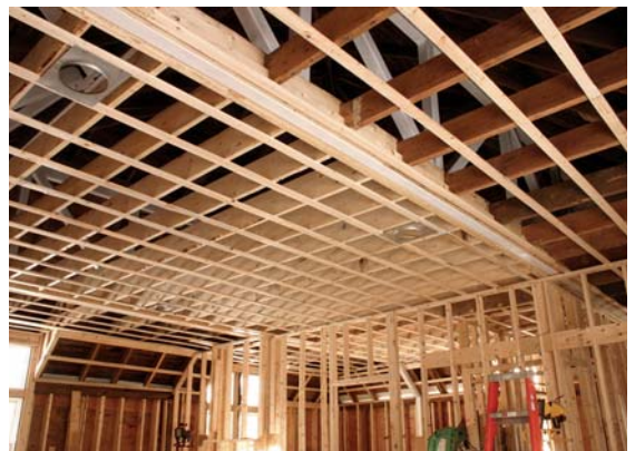
Figure 7. After being jacked to its original elevation, the original roof framing was supported by an engineered tubular steel truss (top and above), which was cut on site and assembled in place (top right), then welded together (center right). The truss (painted white) eliminated the need for collar ties and provided a flat ceiling plane (right).
