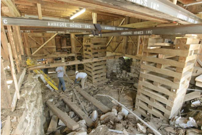
Figure 2. The eight I-beams provided multiple lifting and jacking points. Besides supporting the perpendicular beams, the two 60-foot-long needles picked up the doubled 2x12 ledgers lag-screwed to the wall framing at each end of the barn (above right). Four 40-foot crossmembers caught the ledger along the side walls (right).
