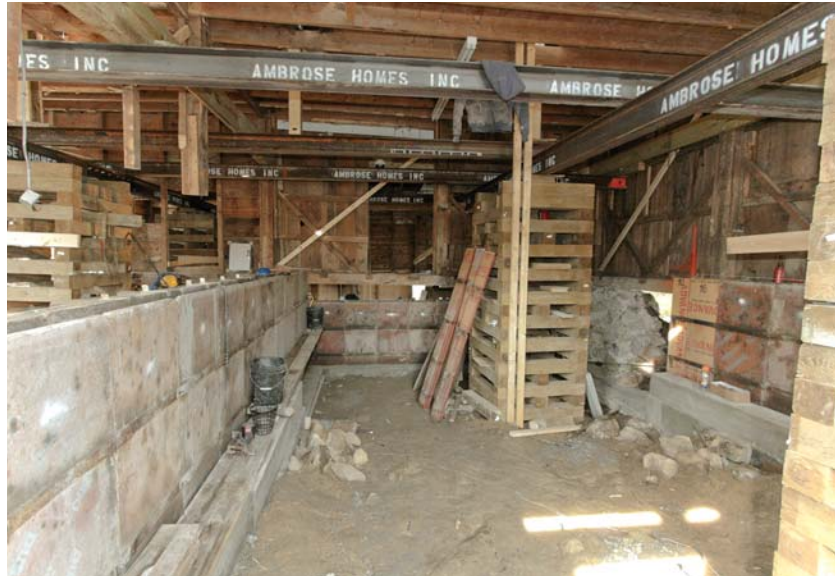
Figure 4. A mini-excavator helped clear the way for the new crawlspace foundation (above left). Reinforced stepped footings and stem walls replaced the original foundation a section at a time (above). Temporarily supporting the original balloon-framed walls on the new foundation ensured stability until the wall framing could be replaced (left).
