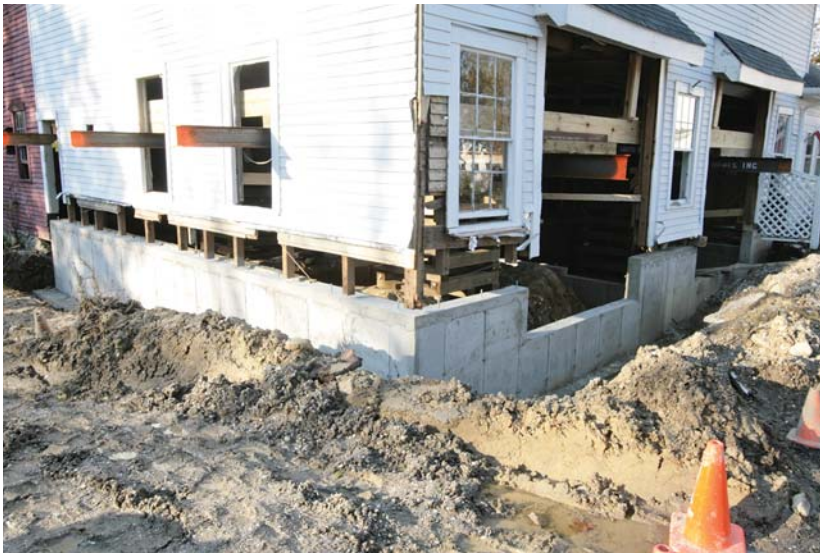
Figure 4. A mini-excavator helped clear the way for the new crawlspace foundation (above left). Reinforced stepped footings and stem walls replaced the original foundation a section at a time (above). Temporarily supporting the original balloon-framed walls on the new foundation ensured stability until the wall framing could be replaced (left).
