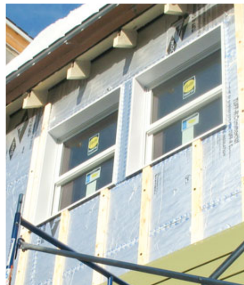
Figure 5. In order to secure the deep exterior jambs needed to cover the double layer of foam, carpenters fastened 2-by blocking around the windows directly against the housewrap (top left). The blocks were covered with \frac{1}{2} -inch-thick foam, then buried beneath the second layer of 2-inch foam, effectively preventing thermal conduction (top right). Stainless fasteners secure the PVC extensions, which were also taped to the foil-faced foam (above photos).
