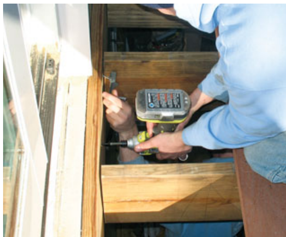
Figure 4. Porch floor joists had to be cut off to allow the insulation board to pass behind (above and top right). The new ledger was attached through the foam into solid framing with structurally rated screws (right).
