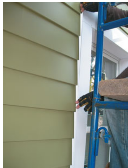
Figure 7. Vertical trim pieces are rabbeted to allow the siding to move horizontally behind them (left). Sawtooth closure strips (below left) plug the gaps where the clapboards run behind the trim (below).
