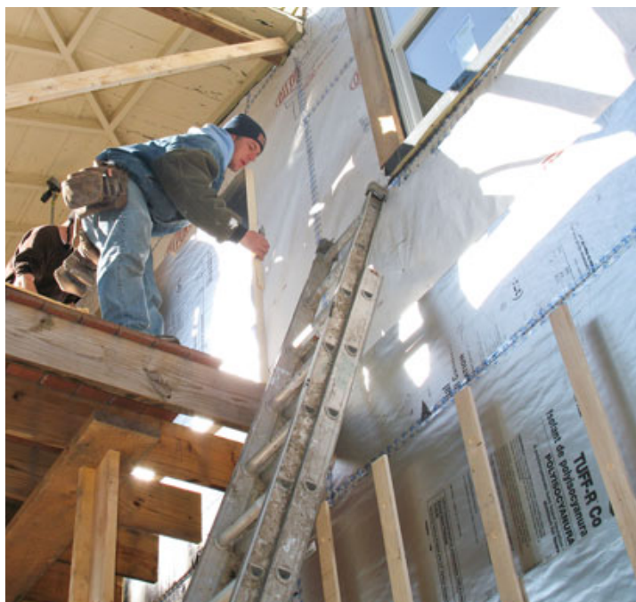
Figure 4. Porch floor joists had to be cut off to allow the insulation board to pass behind (above and top right). The new ledger was attached through the foam into solid framing with structurally rated screws (right).
