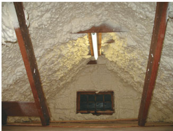
Figure 8. Open-cell spray foam in the attic (top photos) boosted roof R-value to around 60. The benefits of the added insulation were apparent as the job progressed: Ice dams that used to form were gone (left and below).
