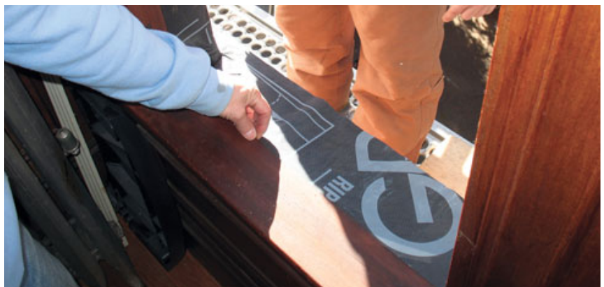
Figure 2. The replacement windows were sized to fit the original double-hung window jambs, which were retained and flashed with a peel-and-stick membrane (left). The interior sills and casing were also preserved (below).
