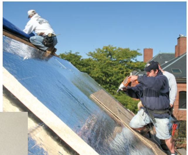
Figure 1. After stripping the existing roofing (above left), the crew installed two staggered layers of 3-inch-thick rigid foam, secured with 10-inch HeadLok screws (inset) driven through the sheathing into the rafters (above).
