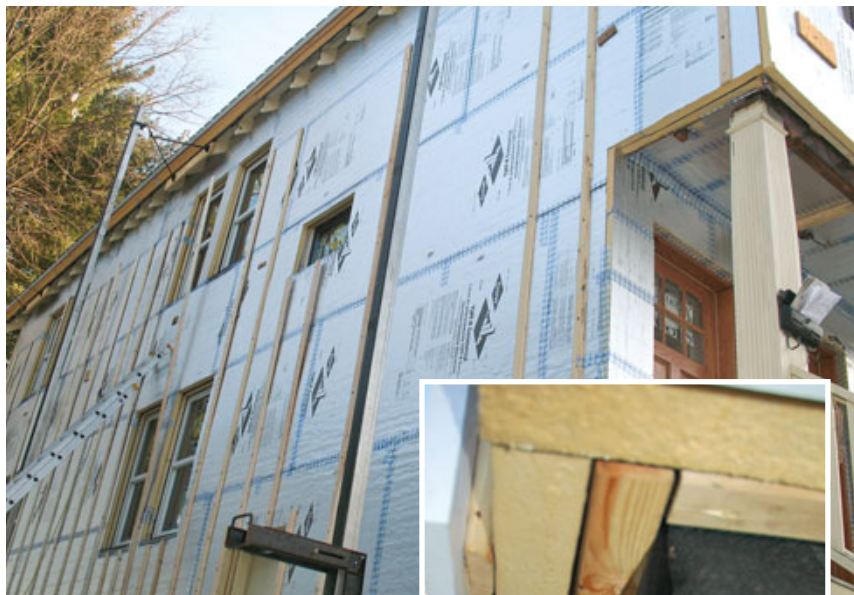
Figure 3. One-by-three strapping screwed to the framing on 16-inch centers holds the double foam layer securely in place (above) and provides a drying and drainage channel behind the siding. Seams on both layers were taped to block air movement. Metal screen (seen hanging, right) keeps insects out of the drainage space.
