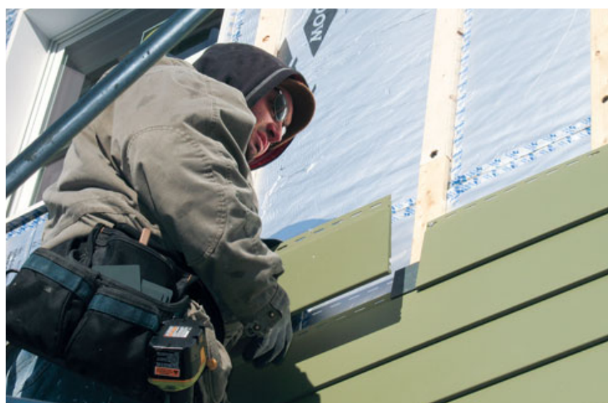
Figure 6. The cellular PVC siding had to be carefully hand-nailed through slots that allow for expansion (top right). Backing plates provide glued reinforcement at butt joints (above and right).
