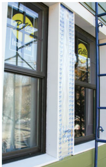
Figure 5. In order to secure the deep exterior jambs needed to cover the double layer of foam, carpenters fastened 2-by blocking around the windows directly against the housewrap (top left). The blocks were covered with \frac{1}{2} -inch-thick foam, then buried beneath the second layer of 2-inch foam, effectively preventing thermal conduction (top right). Stainless fasteners secure the PVC extensions, which were also taped to the foil-faced foam (above photos).
