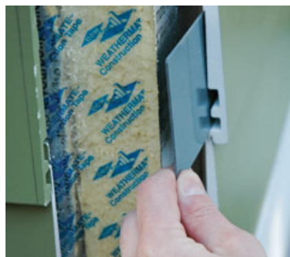
Figure 6. The cellular PVC siding had to be carefully hand-nailed through slots that allow for expansion (top right). Backing plates provide glued reinforcement at butt joints (above and right).
