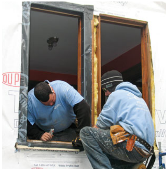
Figure 2. The replacement windows were sized to fit the original double-hung window jambs, which were retained and flashed with a peel-and-stick membrane (left). The interior sills and casing were also preserved (below).
