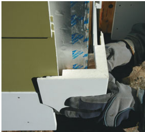
Figure 7. Vertical trim pieces are rabbeted to allow the siding to move horizontally behind them (left). Sawtooth closure strips (below left) plug the gaps where the clapboards run behind the trim (below).
