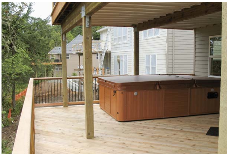
A hot tub weighing 3 tons when full added to the challenge of building an airy deck.
