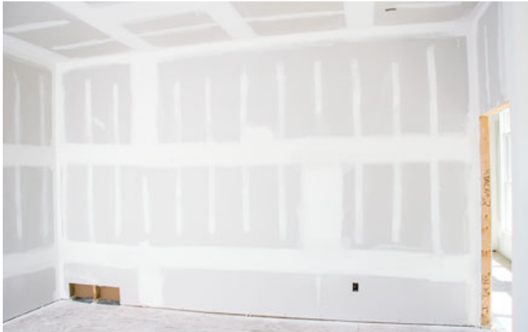
Figure 1. Coating joints and fasteners with joint compound adds different textures and porosities to the paper face of gypsum board (left). Sanding the compounded areas smooth (above) can actually raise the paper's fibers, producing yet another texture.
