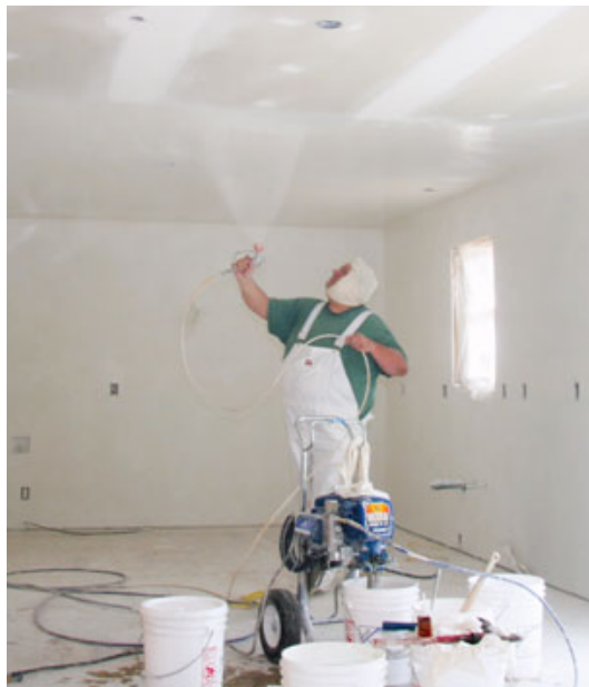
Figure 4. Thick-bodied primer-surfacers are a cost-effective alternative to skim-coating for a Level 5 finish. Applied with an airless sprayer to a 15- to 20-mil thickness, the primer provides a uniform white surface.
