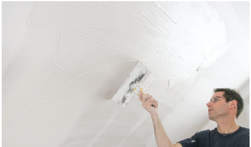
Figure 3. To add a skim coat, the author mixes up a bucket of watered-down joint compound (top left) and applies it to the drywall with a 1/2-inch-nap paint roller (top right). He removes excess compound with a wide knife (above) before it has a chance to dry, then lightly sands the entire surface before priming.
