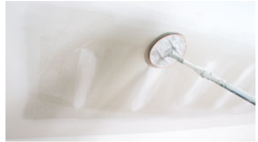
Figure 1. Coating joints and fasteners with joint compound adds different textures and porosities to the paper face of gypsum board (left). Sanding the compounded areas smooth (above) can actually raise the paper's fibers, producing yet another texture.
