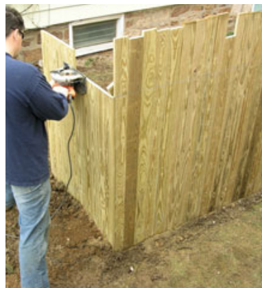
Figure 17. Cutting the slats off in place ensures a straight, continuous line.
