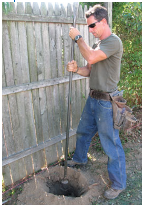
Figure 5. An auger mounted on a sub-compact loader makes quick work of post holes (top). Loose dirt left by the auger can be compacted with the flat end of a digging bar (bottom). Skip this step and your posts may settle or, even worse, lean.
