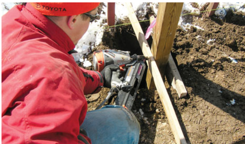
Figure 6. Temporary braces fastened to the posts at grade help to steady them and provide a reference that aids in setting the posts square to the line of the fence.
