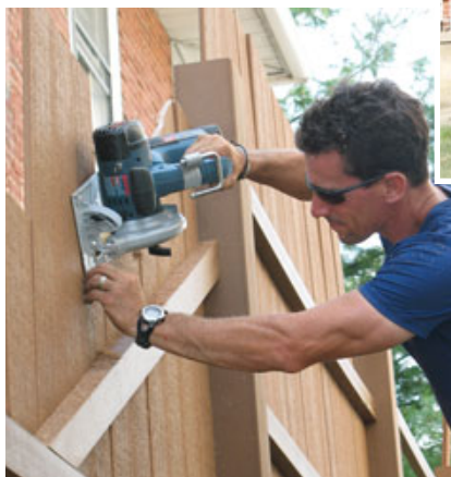
Figure 13. A “swoop” makes for an elegant termination (above). Avoid complicated layout by using cap stock to establish the swoop (far left). Setting the blade to just make it through the slats allows the circular saw to cut wide-radius curves (left).
