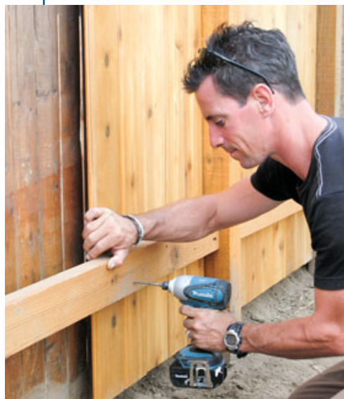
Figure 11. Screwing through the rail into the back of the slats isn't the first approach most carpenters would take, but here, with zero clearance to the neighboring fence, it was the only way.
