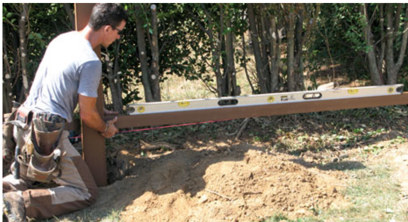
Figure 12. The FenceScape rails are fastened to the post with brackets and screws, helping to brace the post before it's set in concrete.
