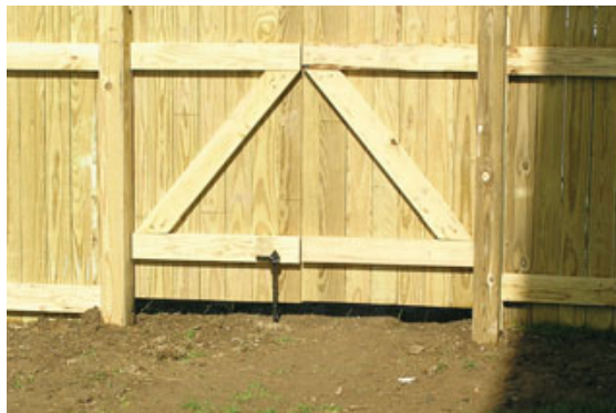
Figure 18. The key to gates that don't sag is a Z-shaped support structure.
