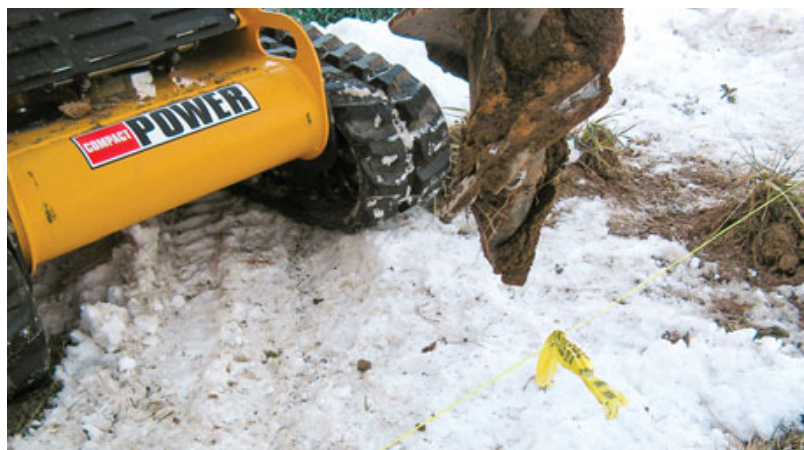
Figure 14. When speed counts more than a precise post layout, mark the approximate post locations on the string using caution tape, and auger away.
