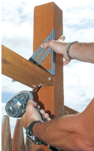
Figure 10. Pocket screws make stout connections. Depending on the material, be sure to soak the holes with stain or end-cut preservative.
