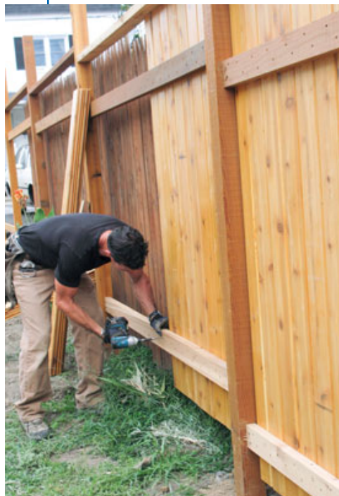
Figure 7. Stepping the fence to match the grade keeps the rails level. Steeper grades require either spacing the posts closer or angling the rails.
