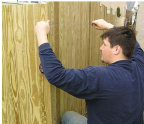
Figure 16. Long runs of fencing may require snapping the cutline in sections to avoid line sag.
