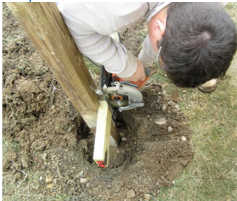
Figure 15. By using longer rails, the author can fasten them to the posts, then cut them to length without measuring. Not having to measure saves a lot of time.
