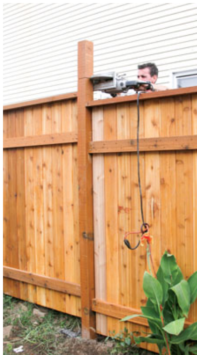
Figure 8. It's difficult to set posts to exactly the right height. Instead, run them tall and cut them to size once the fence is built.
