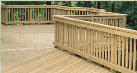
Figure 13. Osmose claims that although its MicroPro wood treatment contains copper, the formulation is no more corrosive than CCA.
