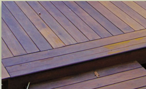
Figure 14. Thermally modified wood, such as this by Cambia Wood, takes on a rich brown color from the manufacturing process.
