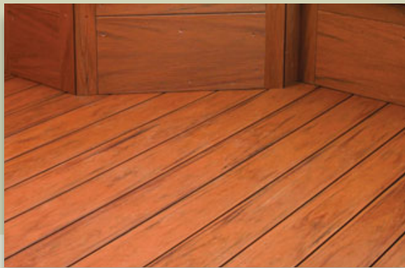
Figure 9. A PVC-coated hybrid, XLM decking comes with a Class A fire rating that should allow its use in wildland-urban interface fire zones.
