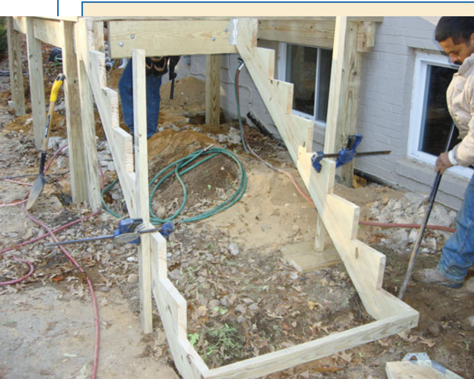
Clamp temporary posts to stringers so the concrete landing can be poured exactly in place.
