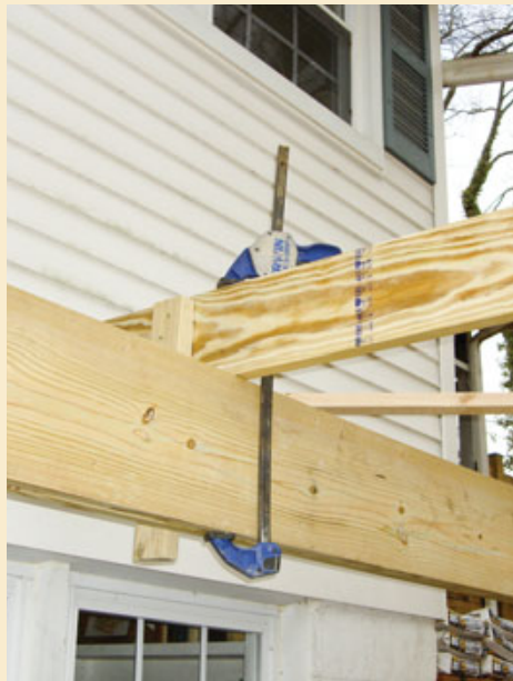
Another way to line up beam members is to clamp them to a perpendicular joist.
