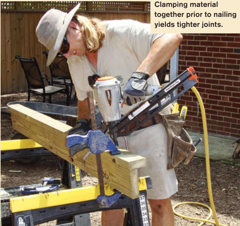
Clamp temporary posts to stringers so the concrete landing can be poured exactly in place.
