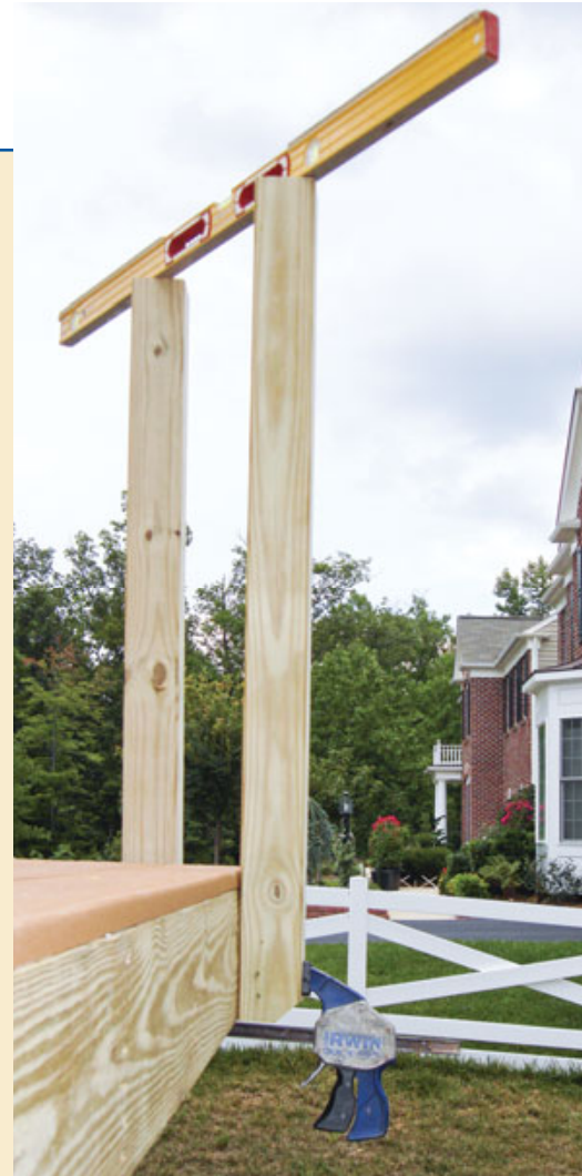
A couple of hammer taps will level out adjacent newels.
