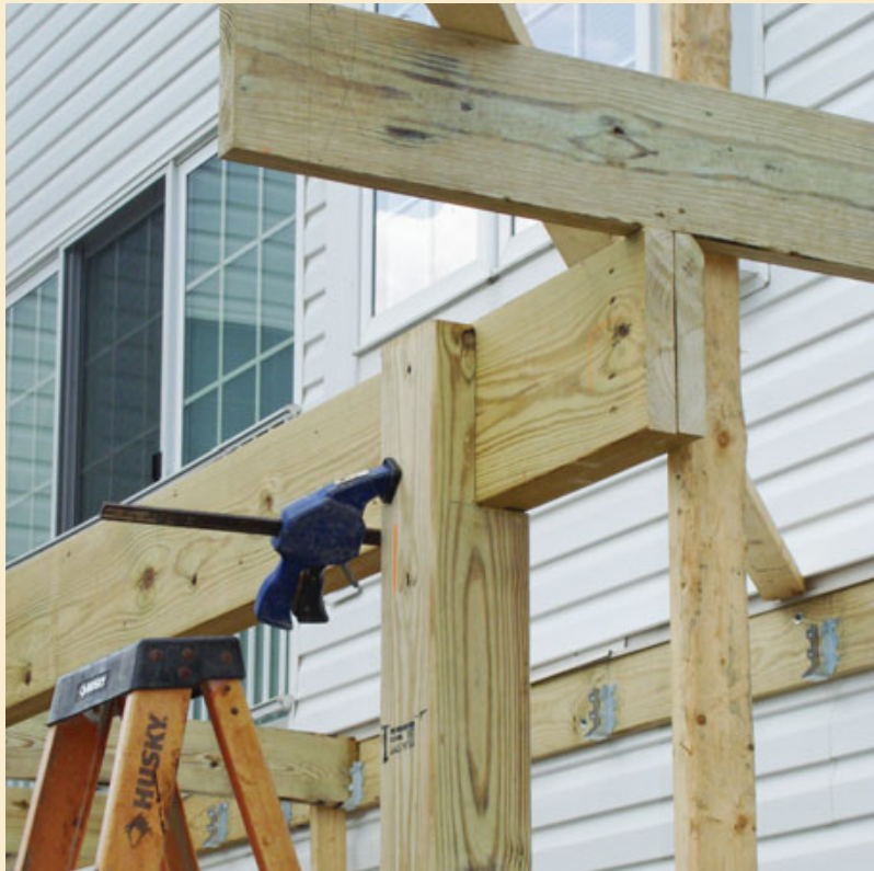
Clamps secure a post and beam prior to drilling and bolting.
