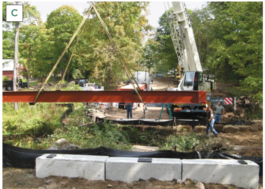
Figure 4. The painted rail cars arrived by truck, along with pressure-treated lumber for the rails and deck. Note the welded brackets on the top flatcar for attaching rail posts (A). The truck backed into place (B), where a large crane stood ready to place the 11,000-pound rail cars onto rubber isolation pads on the concrete abutments (C, D).
