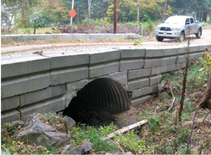
Figure 1. While an open-bottom arch culvert might have worked for the stream crossing, it would have had a greater impact on the stream and was aesthetically less pleasing than the flatcar bridge.
