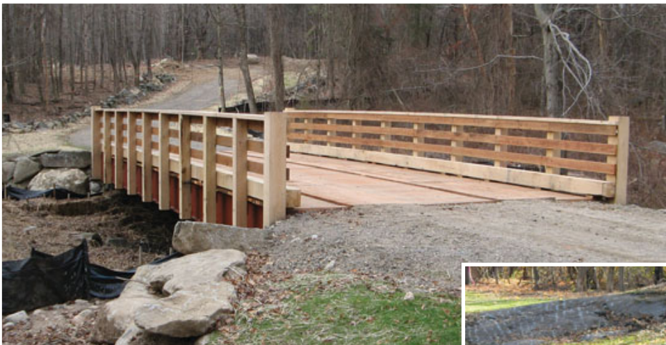
Figure 5. Native red oak 6x6 and 8x8 posts were attached to the predrilled brackets along the sides of the bridge, then the pressure-treated rail was attached. Wood planking and an oak curb completed the project.
