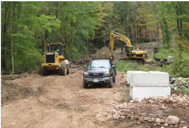
Figure 2. After rough-grading the access to the stream crossing (above), the excavation contractor dug trenches for setting the concrete abutments (right). He leveled the bottoms with stone fill and gravel, then placed a series of interlocking pre-cast blocks (far right).
