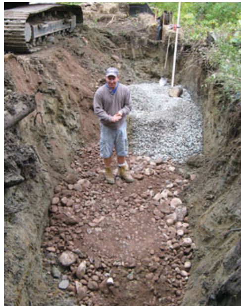
Figure 2. After rough-grading the access to the stream crossing (above), the excavation contractor dug trenches for setting the concrete abutments (right). He leveled the bottoms with stone fill and gravel, then placed a series of interlocking pre-cast blocks (far right).
