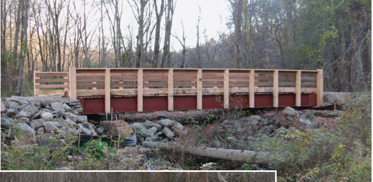
Figure 5. Native red oak 6x6 and 8x8 posts were attached to the predrilled brackets along the sides of the bridge, then the pressure-treated rail was attached. Wood planking and an oak curb completed the project.
