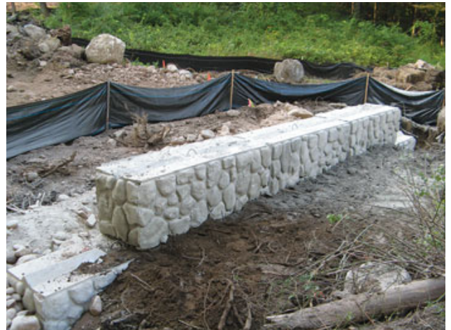
Figure 3. At grade, the abutments transition from plain rectangular blocks to blocks with a precast faux-stone face. Note the silt fences in the background.
