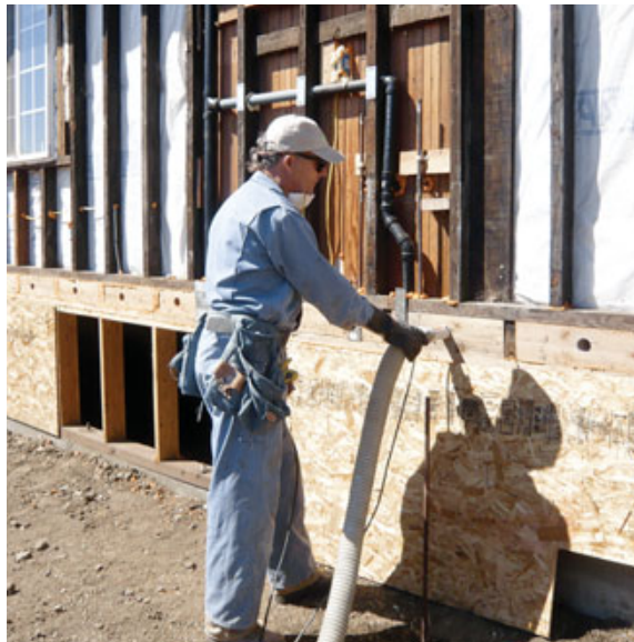
Figure 6. The floor was insulated with dense-pack cellulose blown through holes in the joist blocking. To ensure the cavities were completely filled, the insulator connected a PVC pipe to the hose and began blowing from the far end of the bay (left), withdrawing the pipe as he went (below).
