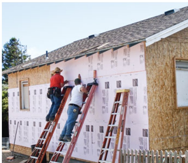
Figure 7. A one-inch layer of rigid XPS foam covers the wall sheathing, providing added R-value and a thermal break. Flat roof vents and a pair of gable-end vents supply attic ventilation.
