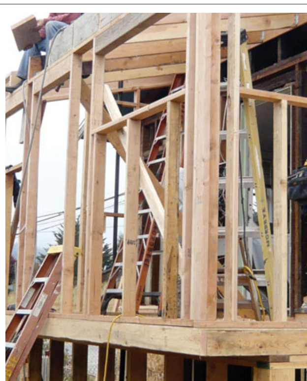
Figure 2. The back laundry room was rebuilt with optimum value engineering (OVE) framing, a method that reduces thermal bridging and saves material. With OVE framing (left) there is 24-inch stud spacing, a single top plate, two-stud corners, right-size headers, and no jack studs. All of the framing in the house was sprayed (above) with Borrada LP, a low-toxicity glycol-borate preservative that kills termites 4 inches into the wood and prevents new infestations — a task made much easier by the additional crawl-space height provided by the new foundation.
