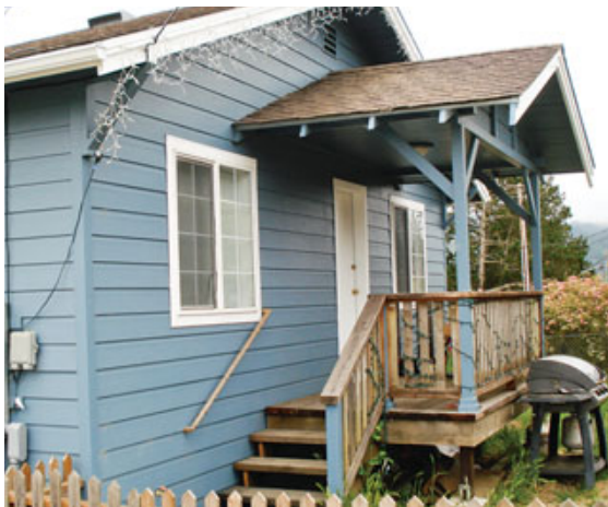
Figure 8. To maintain the continuity of the exterior rigid foam, the small front porch — shown here (left) with the siding applied — was cut free of the structure and then reattached after the foam had been slipped behind it. The back laundry room — a former porch — is fully insulated and lies within the building's thermal envelope (right).
