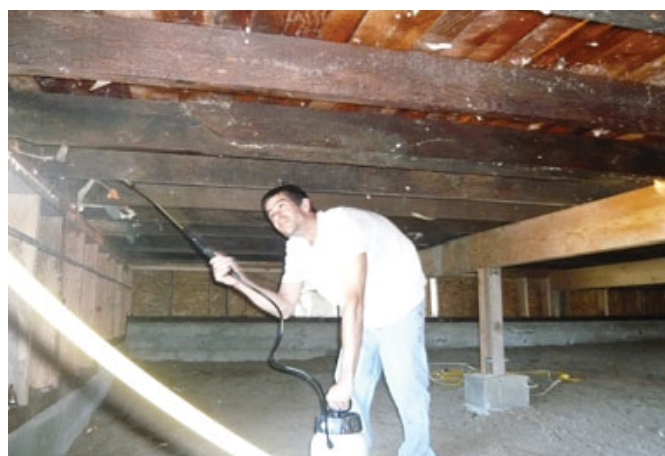
Figure 2. The back laundry room was rebuilt with optimum value engineering (OVE) framing, a method that reduces thermal bridging and saves material. With OVE framing (left) there is 24-inch stud spacing, a single top plate, two-stud corners, right-size headers, and no jack studs. All of the framing in the house was sprayed (above) with Borrada LP, a low-toxicity glycol-borate preservative that kills termites 4 inches into the wood and prevents new infestations — a task made much easier by the additional crawl-space height provided by the new foundation.
