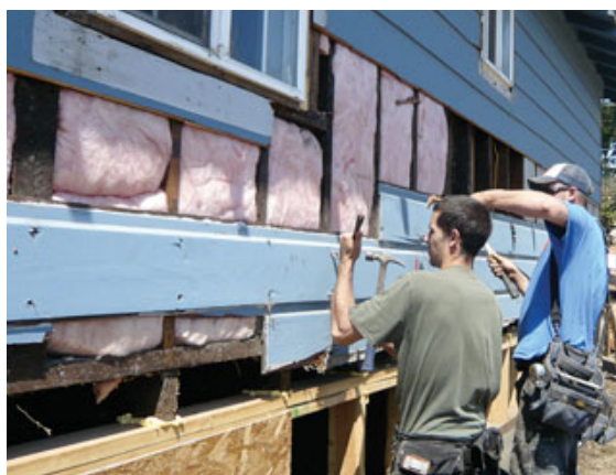
Figure 1. After placing the house on a new foundation and pony walls (above), the crew removed the siding (left) so they could access the stud bays for air-sealing and then install sheathing.
