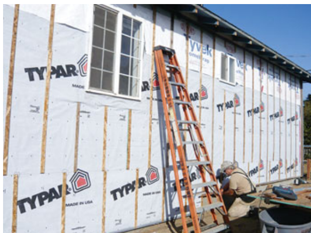
Figure 9. After reinstalling the existing windows, the crew covered the rigid foam with housewrap and vertical battens, which provide an air space and drainage plane behind the siding.
