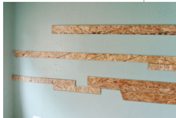
Figure 5. The insulation contractor used the dense-pack method to insulate the newly framed back porch, blowing cellulose through slits in mesh fabric that had been stapled across the studs (left). Where drywall was already up, he blew insulation through holes in the sheathing (below left). The crew screwed temporary braces (below) across the existing drywall to keep it from popping off while cellulose was being packed into the wall.
