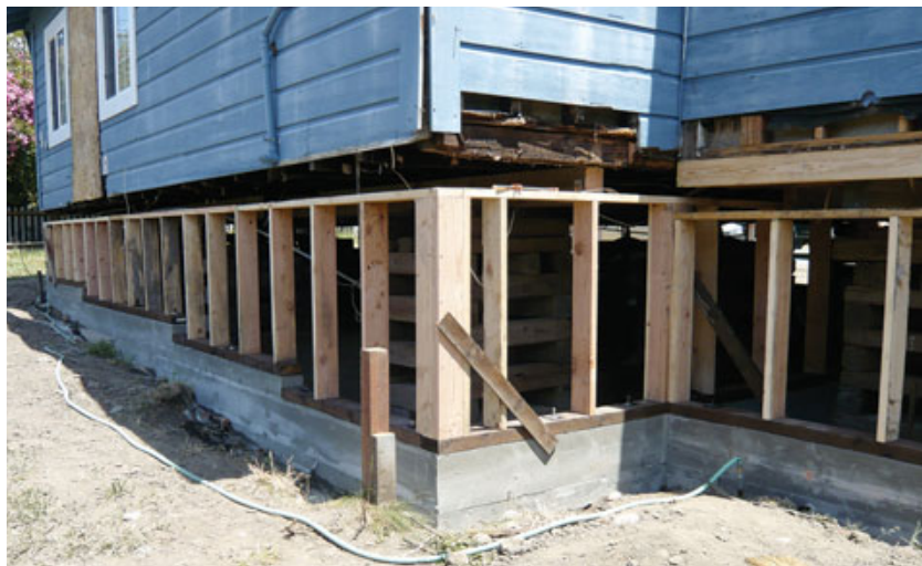
Figure 1. After placing the house on a new foundation and pony walls (above), the crew removed the siding (left) so they could access the stud bays for air-sealing and then install sheathing.
