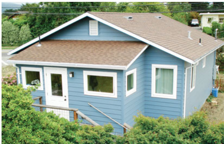
Figure 8. To maintain the continuity of the exterior rigid foam, the small front porch — shown here (left) with the siding applied — was cut free of the structure and then reattached after the foam had been slipped behind it. The back laundry room — a former porch — is fully insulated and lies within the building's thermal envelope (right).
