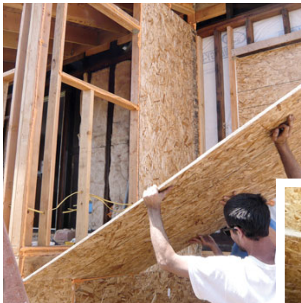
Figure 4. The carpenters installed the sheathing over beads of fresh spray foam (above), which expanded to fill any gaps (above right). The seams in the OSB on the underside of the floor joists (right) were sealed with strips of paper drywall tape laid into a coating of duct mastic.
