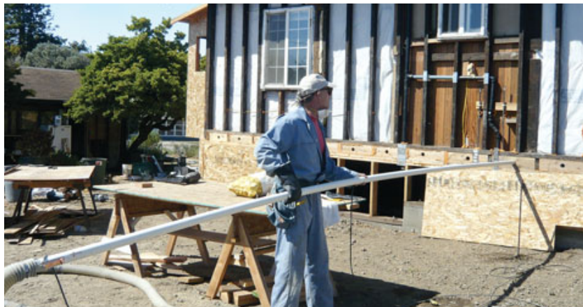
Figure 6. The floor was insulated with dense-pack cellulose blown through holes in the joist blocking. To ensure the cavities were completely filled, the insulator connected a PVC pipe to the hose and began blowing from the far end of the bay (left), withdrawing the pipe as he went (below).
