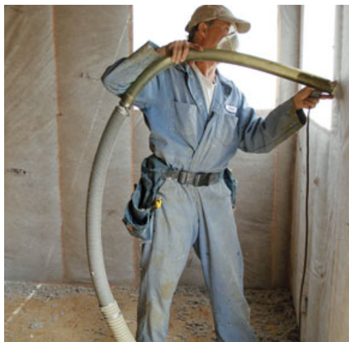
Figure 5. The insulation contractor used the dense-pack method to insulate the newly framed back porch, blowing cellulose through slits in mesh fabric that had been stapled across the studs (left). Where drywall was already up, he blew insulation through holes in the sheathing (below left). The crew screwed temporary braces (below) across the existing drywall to keep it from popping off while cellulose was being packed into the wall.
