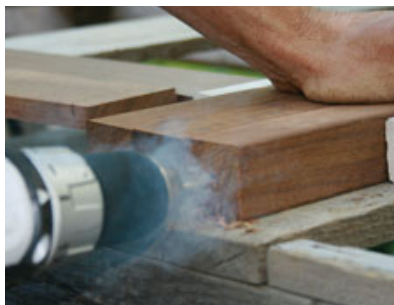
Figure 5. Drilling hardwood generates a lot of heat. Be careful not to touch hot bits to your skin or to any standing water (it can cause the bit to break).
