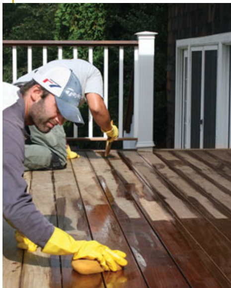
Figure 8. A two-man finishing crew minimizes lap marks. One works the finish between the boards with a brush while the second crew member quickly coats the field using a sponge.
