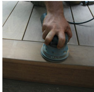
Figure 7. Before finishing hardwood, give it a quick sanding with 80-grit paper in an orbital sander.
