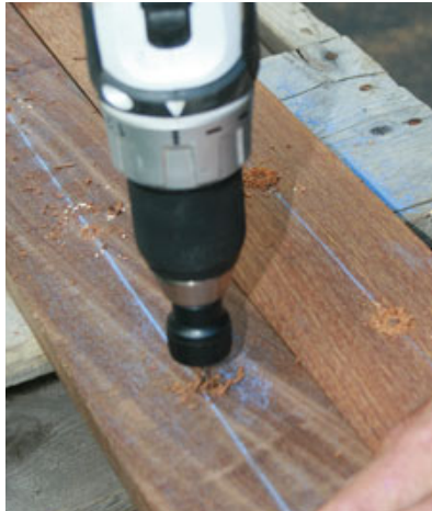
Figure 3. When attaching hardwood with screws, all the holes must be drilled and countersunk.
