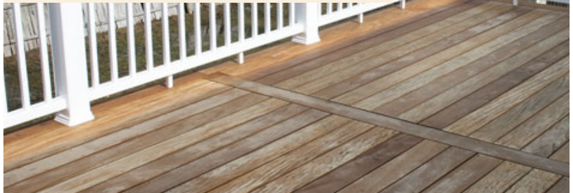
Figure 1. Plan hardwood installations around the material. Picture-framing the outside of the deck hides saw-cut burns on the end grain. Parting boards, that is, boards that run perpendicular to the main deck, add a detail and allow the use of shorter material for the main boards.
