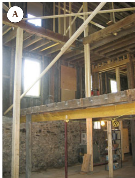
Figure 3. The floor framing was removed in sections and interior bracing installed to stabilize the walls; tall posts supported the floor system above (A). Because the original oak sill was rotting (B), the crew placed a new 2x4 pressure-treated sill on the inner portion of the wide foundation, then set a double-LVL rim joist on top to catch the ends of the new I-joists (C). This approach allowed reframing of the floors to proceed in sections (D).
