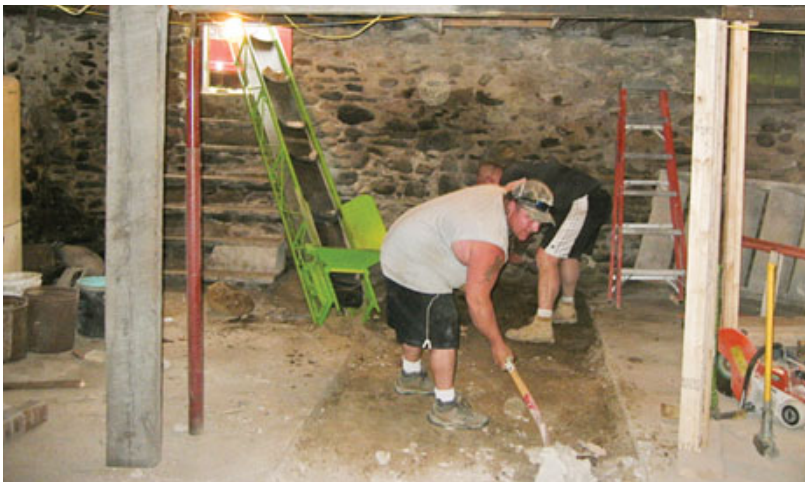
Figure 2. One of the first orders of business was to provide a center bearing wall in the basement. After cutting through the thin slab, the author's crew dug a trench the length of the basement for a new reinforced concrete footing (above). To accommodate the bearing walls for a stairway, the 12-inch-deep by 24-inch-wide footing widens to 5 feet at one end of the basement (right).
