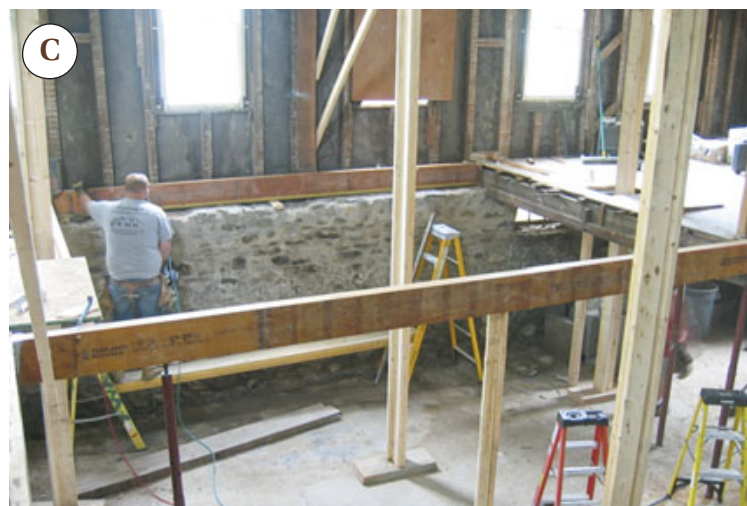
Figure 3. The floor framing was removed in sections and interior bracing installed to stabilize the walls; tall posts supported the floor system above (A). Because the original oak sill was rotting (B), the crew placed a new 2x4 pressure-treated sill on the inner portion of the wide foundation, then set a double-LVL rim joist on top to catch the ends of the new I-joists (C). This approach allowed reframing of the floors to proceed in sections (D).
