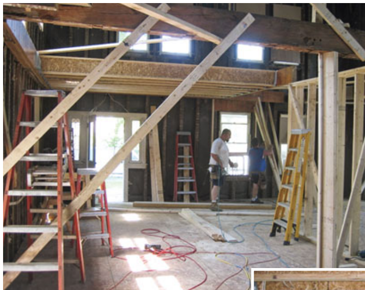
Figure 5. Diagonal braces prevented the exterior walls from spreading as the floors were reframed, a section at a time (above). Meanwhile, carpenters removed the bottom clapboard courses and replaced the rotted sills (above right). After the exterior walls were insulated with closed-cell foam, the author strapped them with 1X2s, shimming or notching as needed to remove the worst irregularities (right).
