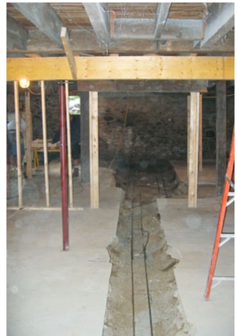
Figure 2. One of the first orders of business was to provide a center bearing wall in the basement. After cutting through the thin slab, the author's crew dug a trench the length of the basement for a new reinforced concrete footing (above). To accommodate the bearing walls for a stairway, the 12-inch-deep by 24-inch-wide footing widens to 5 feet at one end of the basement (right).
