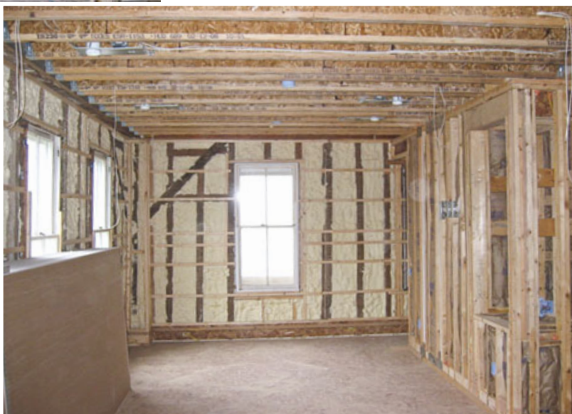
Figure 5. Diagonal braces prevented the exterior walls from spreading as the floors were reframed, a section at a time (above). Meanwhile, carpenters removed the bottom clapboard courses and replaced the rotted sills (above right). After the exterior walls were insulated with closed-cell foam, the author strapped them with 1X2s, shimming or notching as needed to remove the worst irregularities (right).
