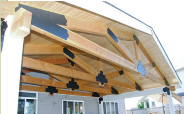
Figure 5. The author designed decorative metal plates to dress up the timber connections in the roof.
