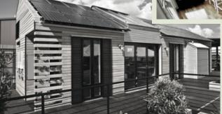
Movable steel shutters provide both shade and highwind protection.
