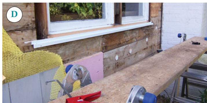
Figure 1. After cutting each sill flush with the sheathing (A) and planing down the tongues on the jambs (B), the author ripped kerfs in the sills (C) to accept a custom-bent aluminum flashing (D). The metal flashings are bedded in sealant and overlap the new layer of 1-inch-thick rigid XPS foam used to wrap the house.
