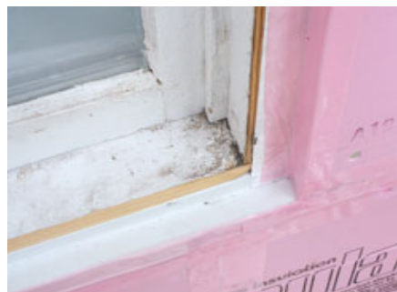
Figure 3. To help make a continuous air barrier, the rigid foam was glued to the flashing tape at the jambs (above left) and to itself at the butt joints (above). The long horizontal tongue-and-groove joints in the rigid foam were left unglued to provide for thermal expansion, but all the joints were taped, and the foam was also taped to the flashings (left).
