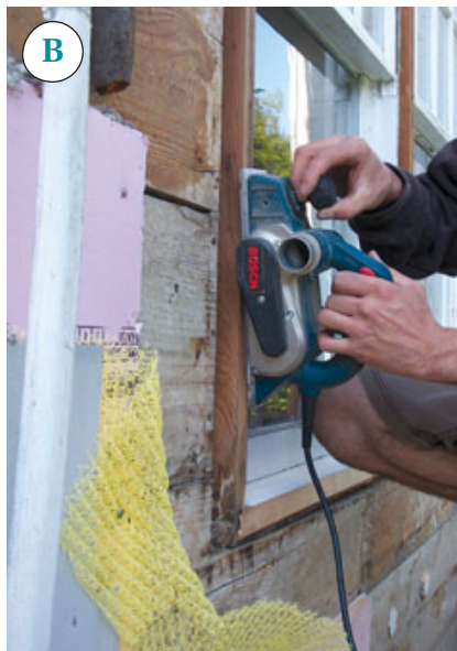
Figure 1. After cutting each sill flush with the sheathing (A) and planing down the tongues on the jambs (B), the author ripped kerfs in the sills (C) to accept a custom-bent aluminum flashing (D). The metal flashings are bedded in sealant and overlap the new layer of 1-inch-thick rigid XPS foam used to wrap the house.
