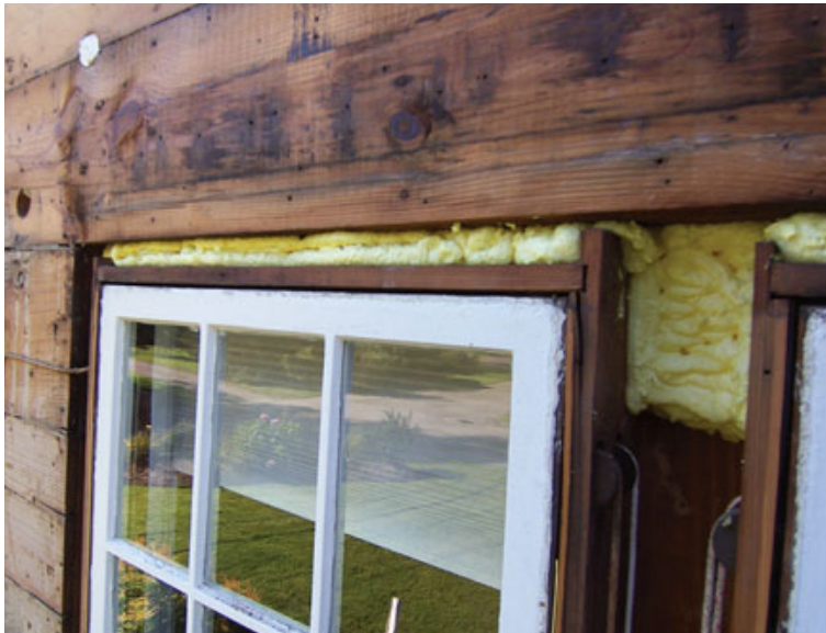
Figure 2. The author insulated around the jambs and in the sash-weight pockets with a combination of rigid and spray foam (above), then flashed the jambs to the sheathing with self-adhering flashing tape (right).
