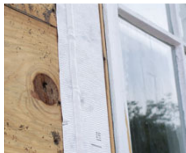
Figure 2. The author insulated around the jambs and in the sash-weight pockets with a combination of rigid and spray foam (above), then flashed the jambs to the sheathing with self-adhering flashing tape (right).
