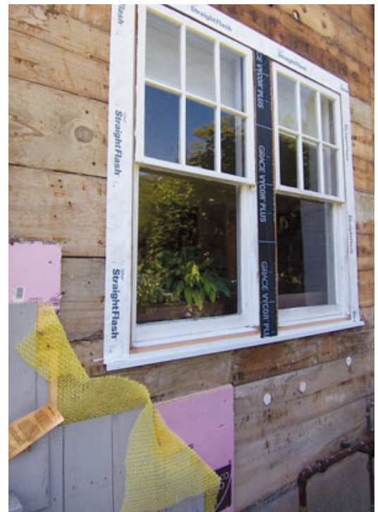
Figure 2. The author insulated around the jambs and in the sash-weight pockets with a combination of rigid and spray foam (above), then flashed the jambs to the sheathing with self-adhering flashing tape (right).
