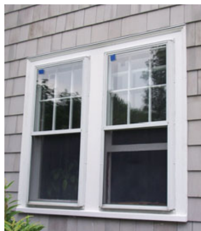
Figure 5. To allow for water and air movement between the shingles and the foam, the shingles were installed over Home Slicker, a 1/4-inch-thick nylon mesh (above left). Screening over windows (above right) and at other terminations is needed to keep insects out. When painted, the new windows (right) look nearly identical to the originals.
