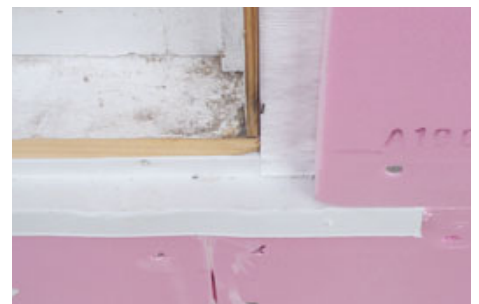
Figure 3. To help make a continuous air barrier, the rigid foam was glued to the flashing tape at the jambs (above left) and to itself at the butt joints (above). The long horizontal tongue-and-groove joints in the rigid foam were left unglued to provide for thermal expansion, but all the joints were taped, and the foam was also taped to the flashings (left).
