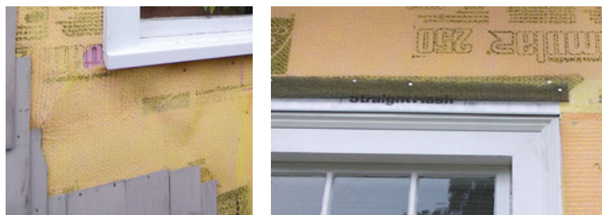
Figure 5. To allow for water and air movement between the shingles and the foam, the shingles were installed over Home Slicker, a 1/4-inch-thick nylon mesh (above left). Screening over windows (above right) and at other terminations is needed to keep insects out. When painted, the new windows (right) look nearly identical to the originals.
