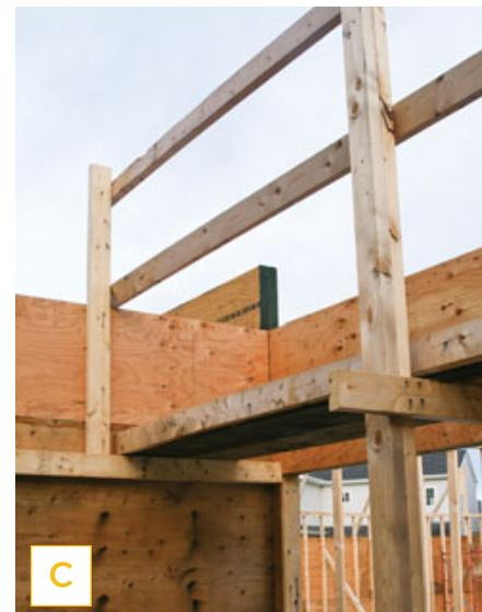
Previously, the author paid thousands of dollars in OSHA fines for fall-protection violations on this job site, because his crew was walking the top plates to set trusses and accessing the plate using stepladders. Now the crew sets up OSHA-compliant scaffolding with railings and toeboards at the building eaves (A) and uses extension ladders to access the staging (B). At inside corners, the author uses the building's side walls to support the staging planks (C).
