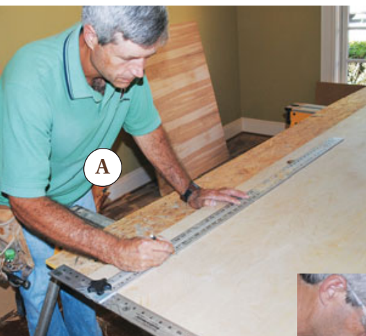
Figure 1. When laying out the design, the author usually mimics the stile and rail dimensions of a traditional frame-and-panel door (A). The panels are assembled with glue and 1½-inch-long 23-gauge headless pins (B), then glued (C) and pinned to the door slab following the layout marks (D).
