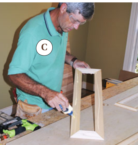
Figure 1. When laying out the design, the author usually mimics the stile and rail dimensions of a traditional frame-and-panel door (A). The panels are assembled with glue and 1½-inch-long 23-gauge headless pins (B), then glued (C) and pinned to the door slab following the layout marks (D).
