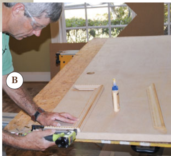
Figure 1. When laying out the design, the author usually mimics the stile and rail dimensions of a traditional frame-and-panel door (A). The panels are assembled with glue and 1½-inch-long 23-gauge headless pins (B), then glued (C) and pinned to the door slab following the layout marks (D).
