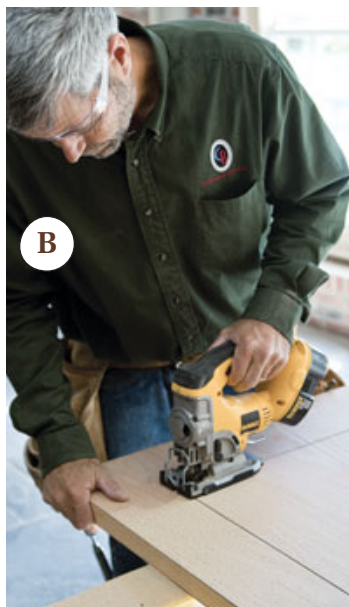
Figure 3. To cut the openings for glass panels in solid-core doors, the author first plunge-cuts with a track saw (A), then finishes up the corners with a jigsaw (B), leaving a clean cutout with square corners (C).
