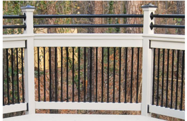
Figure 6. The added height and hard-to-grip surfaces on this railing are meant to keep cats on the deck and out of the reach of local coyotes.
