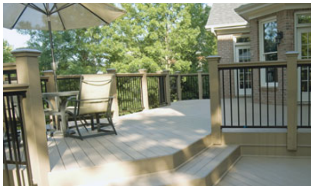
Figure 1. Azek rail caps, painted cedar posts, locally sourced welded railing sections, and Maine Ornamental post caps form a railing designed to meet a specific height requirement.
