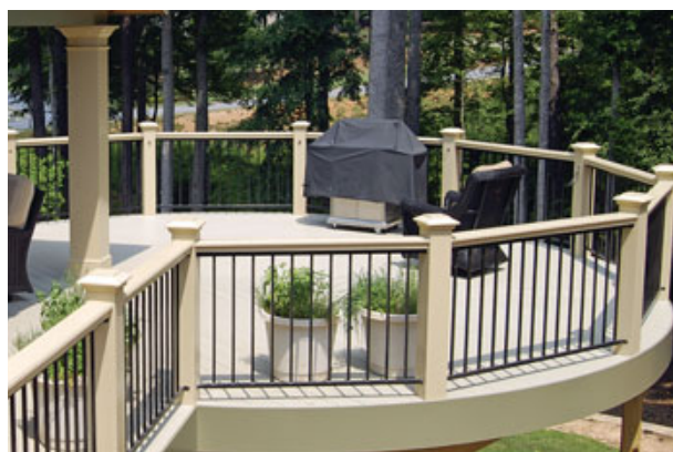
Figure 2. Although painting a wood railing system to match the home's colors might seem to invite frequent maintenance, proper preparation and high-quality paint can create a long-lasting job.
