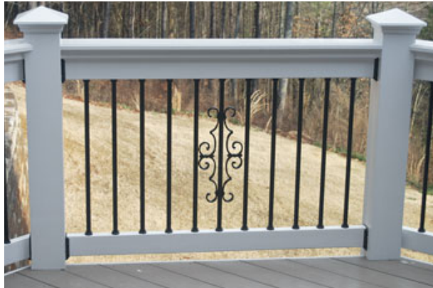
Figure 5. Heavy 6x6 cedar posts, a traditional Deckorators PVC rail cap, and Maine Ornamental post caps frame a view kept relatively unobstructed by the use of thin aluminum balusters.
