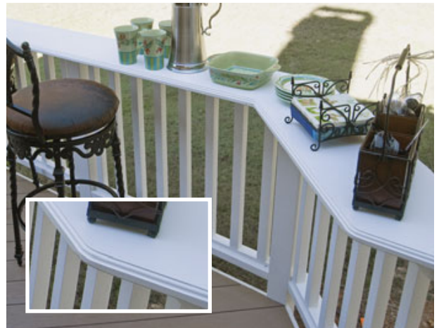
Figure 7. The wide ledge on this railing creates a bar and seating space away from the table area, which improves a deck's ability to host parties. Note the routed profile (inset).
