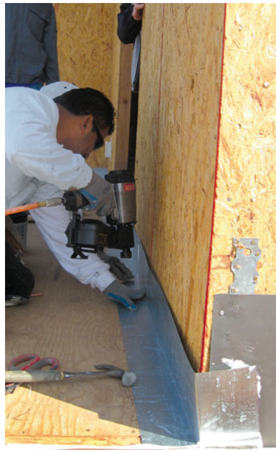
Figure 2. L-shaped flashings are installed at the transition between deck and wall. A slit in the bottom leg of this piece allows it to be folded into the corner (above left). All laps are sealed with double beads of polyurethane caulk (above right), and the flanges are nailed to the deck and wall (right). When the building paper is installed, it will lap the flashing shingle-style.
