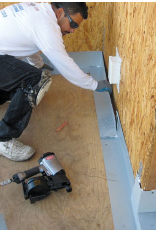
Figure 2. L-shaped flashings are installed at the transition between deck and wall. A slit in the bottom leg of this piece allows it to be folded into the corner (above left). All laps are sealed with double beads of polyurethane caulk (above right), and the flanges are nailed to the deck and wall (right). When the building paper is installed, it will lap the flashing shingle-style.
