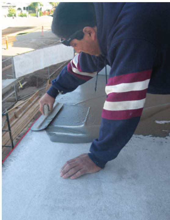
Figure 6. Long exposure to sunlight will damage the acrylic resin membrane, so it is protected under a thin layer of the same polymer cement that was used to cover the lath.
