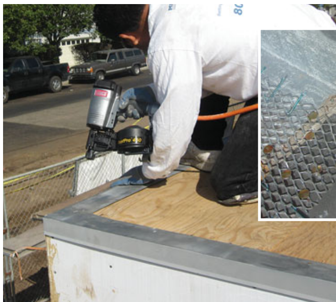
Figure 3. Since the deck slopes to the exterior, the gravel stop is installed from low to high so that the pieces lap shingle-style. Where the deck meets the wall of the building, the gravel stop butts the L-shaped flashing and laps the Z-flashing below (inset).
