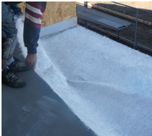
Figure 5. When the first layer of cement has cured, it is covered with overlapping sheets of fiberglass matting (left) and then coated with acrylic resin (right). The resin soaks through and bonds the mat to the substrate, then cures to form a continuous waterproof membrane. It's important to lap the resin onto the vertical leg of the wall flashing.
