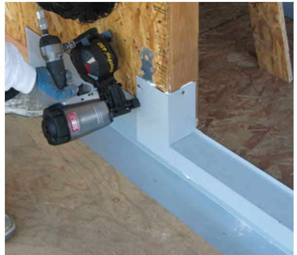
Figure 1. After installing an L-shaped flashing under the door opening, a waterproofing specialist applies polyurethane sealant to the lip of a two-piece door pan (above left). The first piece is installed in the opening and nailed to the trimmers (above). A second piece laps onto the first near the center of the opening. The lap won't leak, because it contains beads of sealant (far left). To avoid penetrations through the bottom of the pan, the crew uses a sprung board to clamp it in place until the sealant below it cures (left).
