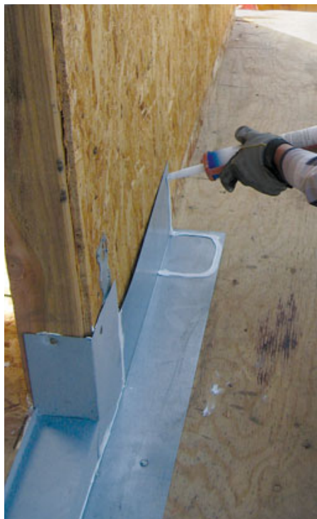
Figure 2. L-shaped flashings are installed at the transition between deck and wall. A slit in the bottom leg of this piece allows it to be folded into the corner (above left). All laps are sealed with double beads of polyurethane caulk (above right), and the flanges are nailed to the deck and wall (right). When the building paper is installed, it will lap the flashing shingle-style.
