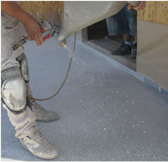
Figure 7. After the second layer of polymer cement cures, the deck can be finished — in this case with a spray-applied texture (left) troweled flat shortly after application to leave a knockdown finish (above).
