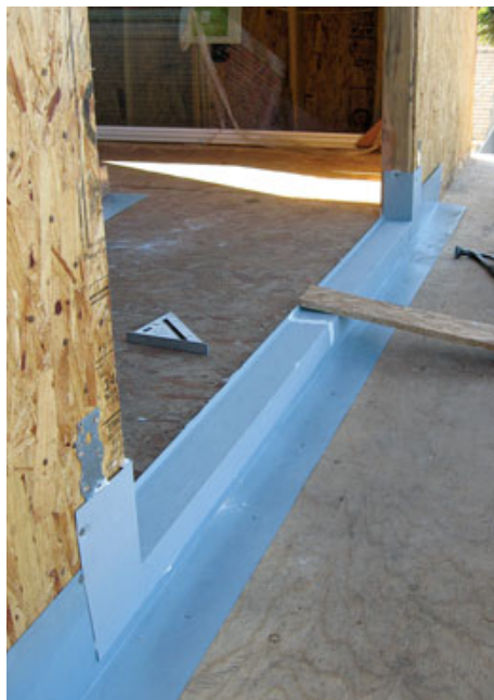
Figure 1. After installing an L-shaped flashing under the door opening, a waterproofing specialist applies polyurethane sealant to the lip of a two-piece door pan (above left). The first piece is installed in the opening and nailed to the trimmers (above). A second piece laps onto the first near the center of the opening. The lap won't leak, because it contains beads of sealant (far left). To avoid penetrations through the bottom of the pan, the crew uses a sprung board to clamp it in place until the sealant below it cures (left).
