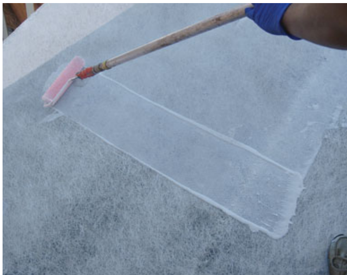
Figure 5. When the first layer of cement has cured, it is covered with overlapping sheets of fiberglass matting (left) and then coated with acrylic resin (right). The resin soaks through and bonds the mat to the substrate, then cures to form a continuous waterproof membrane. It's important to lap the resin onto the vertical leg of the wall flashing.
