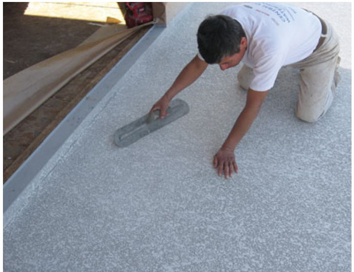
Figure 7. After the second layer of polymer cement cures, the deck can be finished — in this case with a spray-applied texture (left) troweled flat shortly after application to leave a knockdown finish (above).
