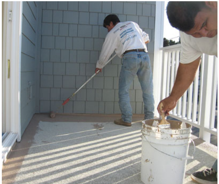
Figure 8. The texture is coated with pigmented concrete sealer, which dries to form a tough walkable surface. Because this deck (above) was finished before the exterior trim was complete, it will require protection while the building paper and siding are installed. More typically, the texture and sealer are applied at the very end of the project (right).
