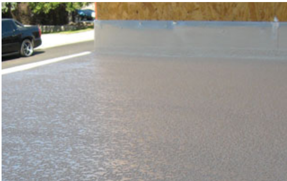
Figure 8. The texture is coated with pigmented concrete sealer, which dries to form a tough walkable surface. Because this deck (above) was finished before the exterior trim was complete, it will require protection while the building paper and siding are installed. More typically, the texture and sealer are applied at the very end of the project (right).
