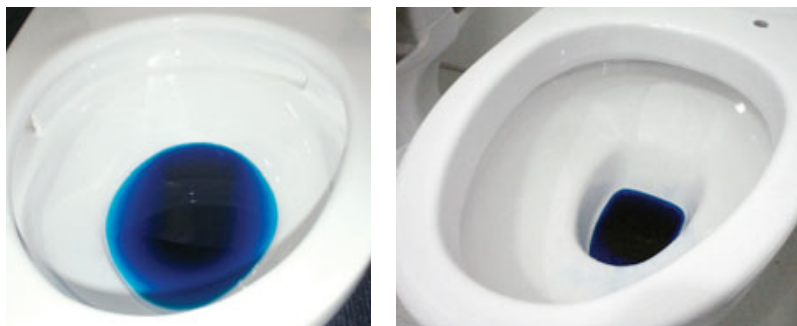
Figure 3. Siphoning toilets tend to stay clean because the water spot — the area of the water inside the bowl — is large enough to keep solids away from the porcelain (left). A wash-down model typically requires frequent brushing because its water spot is too small (right) to keep solids off the bowl.
