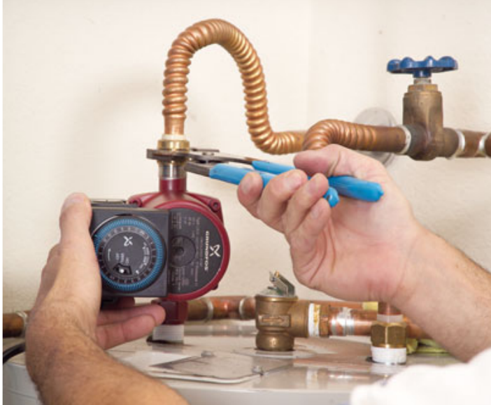
Figure 1. Whole-house hot-water circulation systems use a pump to move cooled water in the hot-water supply line back to the water heater. Closed-loop systems have dedicated return lines (right), but there are also some open-loop systems (above) with special manifolds that allow the cold-water supply to be used as the return line. The pumps shown here are equipped with timers that limit operation to specified periods of demand.
