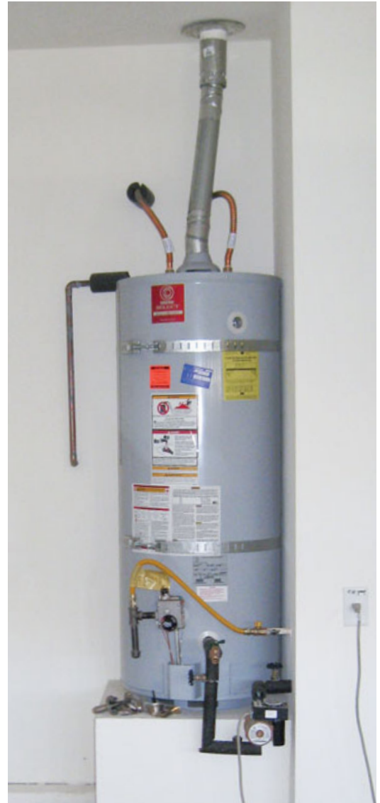
Figure 1. Whole-house hot-water circulation systems use a pump to move cooled water in the hot-water supply line back to the water heater. Closed-loop systems have dedicated return lines (right), but there are also some open-loop systems (above) with special manifolds that allow the cold-water supply to be used as the return line. The pumps shown here are equipped with timers that limit operation to specified periods of demand.
