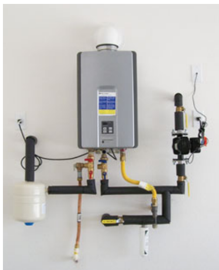
Figure 5. Unlike traditional whole-house circulation systems, on-demand pumps can be used with tankless water heaters without voiding the manufacturer’s warranty. The author uses a \frac{3}{4} -inch hot-water return line and increases the pump size to make sure there is enough flow to activate the burner and to account for friction losses within the heater itself.
