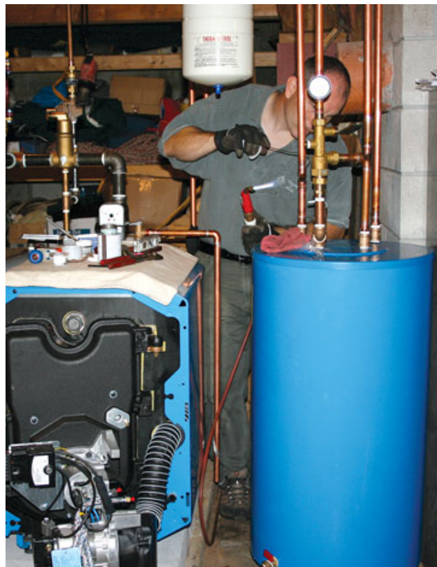
Figure 6. As part of the system upgrade, the author installed new circulator pumps and expansion tanks (left) and an indirect-fired domestic hot-water storage tank (above).
