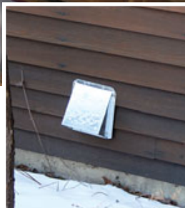
Figure 5. Outside combustion air flows through flexible metal duct (top) and 4-inch-diameter rigid duct to the rear of the boiler (left). The screened air-inlet fitting on the outside wall is protected by a metal cap (inset).
