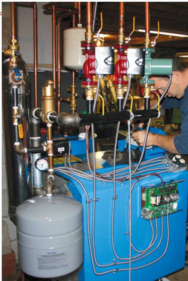
Figure 6. As part of the system upgrade, the author installed new circulator pumps and expansion tanks (left) and an indirect-fired domestic hot-water storage tank (above).
