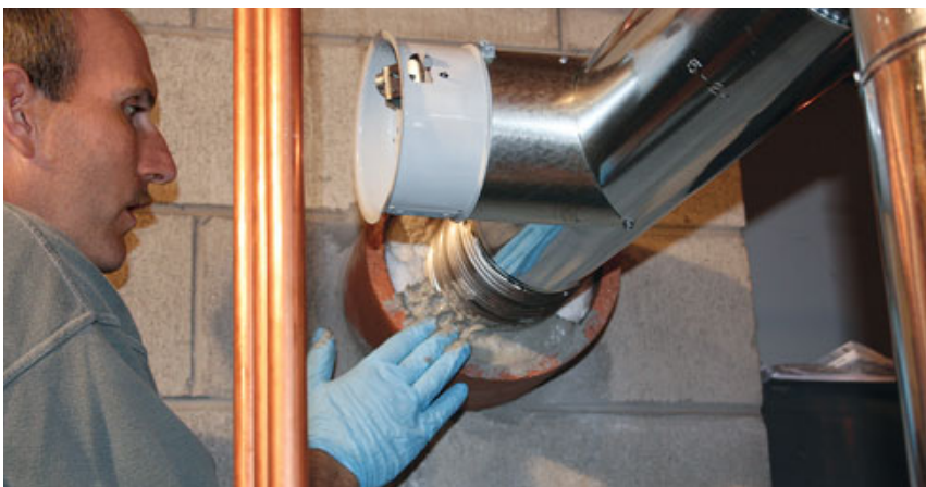
Figure 1. The Buderus G125BE noncondensing boiler can be vented either horizontally or vertically but needs a maximum 5-inch-diameter chimney liner when vented into an oversized masonry chimney flue (top left). At the top, the liner's cap is set in sealant and screwed in place with masonry screws (top right). At the base, the author packs the cavity between the new liner and old flue with mineral wool insulation and seals the opening with refractory cement (above).
