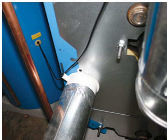
Figure 5. Outside combustion air flows through flexible metal duct (top) and 4-inch-diameter rigid duct to the rear of the boiler (left). The screened air-inlet fitting on the outside wall is protected by a metal cap (inset).
