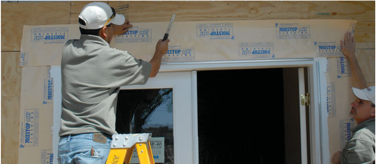
Figure 8. The top flashing laps over the upper nailing flange and is installed after the door is in place (above). Housewrap can be installed either before or after the door unit (left).
