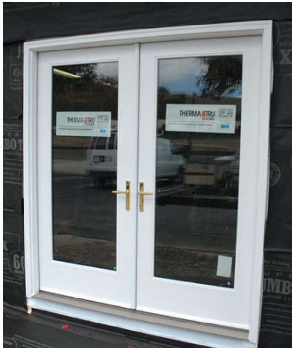
Figure 8. The top flashing laps over the upper nailing flange and is installed after the door is in place (above). Housewrap can be installed either before or after the door unit (left).
