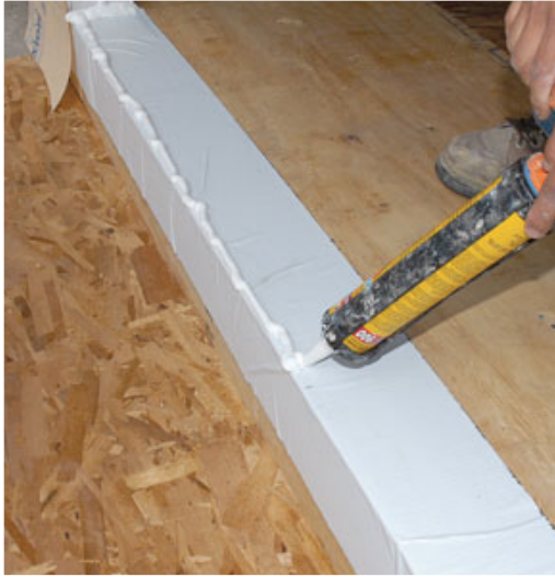
Figure 4. In the barrier method, polyurethane sealant is applied in two continuous \frac{5}{8} -inch-diameter beads all the way across the door pan and 6 inches up both trimmers, one toward the front of the rough opening and one toward the rear (left). In the drainage method, the sealant is applied in elongated triangles, with a 2- to 3-inch gap in the center to allow water to escape (below left). An L-shaped metal dam embedded in sealant and fastened to the floor after the door is installed directs water toward the drainage gap (below right).
