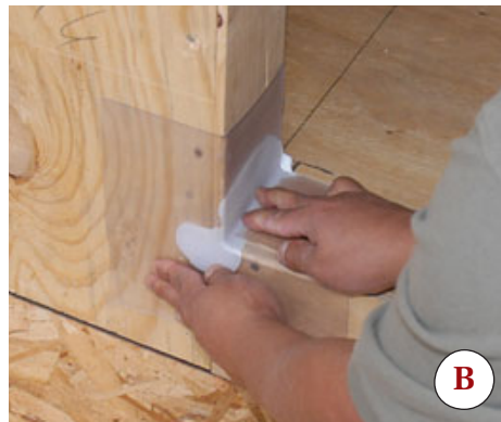
Figure 3. A pair of compatible flexible corner flashings (A) set in beads of sealant (B) are used in conjunction with 12-inch-wide peel-and-stick flashing (C,D) to form a membrane pan. Strips of 9-inch-wide side flashing complete the assembly (E).
