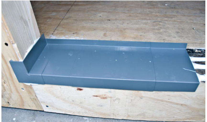
Figure 2. Both one-piece metal door pans (top) and multipiece plastic door pans (above) should be fully bedded in a high-quality polyurethane sealant, not silicone caulk. Membrane pans should always be used with compatible flexible corners (left) and sealants from the same manufacturer; many plasticized sealants are incompatible with peel-and-stick flashings.
