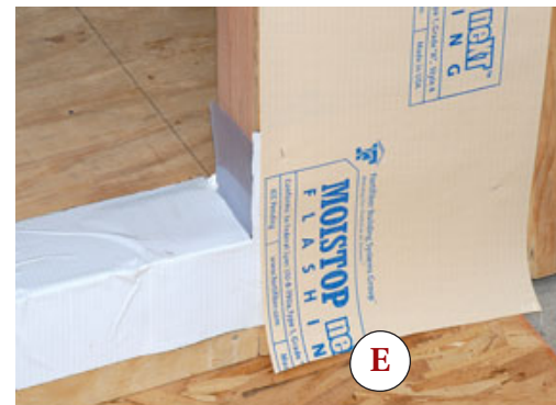
Figure 3. A pair of compatible flexible corner flashings (A) set in beads of sealant (B) are used in conjunction with 12-inch-wide peel-and-stick flashing (C,D) to form a membrane pan. Strips of 9-inch-wide side flashing complete the assembly (E).
