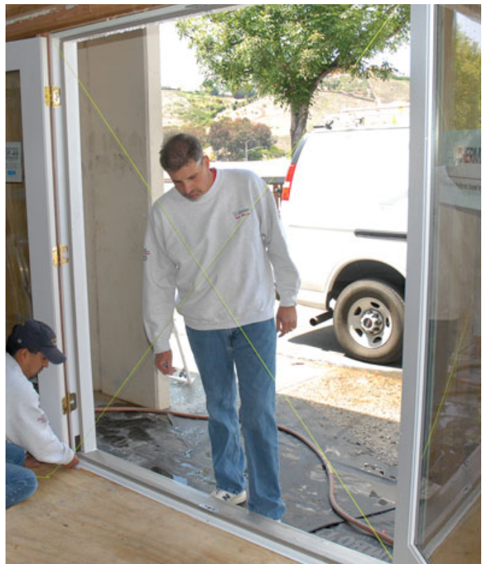
Figure 7. The most accurate way to check if a rough opening or installed door is plumb is with a laser (above), but the easiest way to check for a cross-legged opening or door is with a pair of crisscrossed strings (right). The strings should touch gently in the center.
