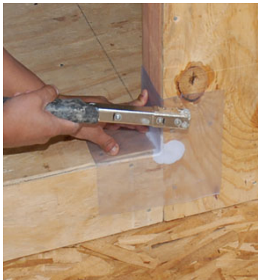
Figure 2. Both one-piece metal door pans (top) and multipiece plastic door pans (above) should be fully bedded in a high-quality polyurethane sealant, not silicone caulk. Membrane pans should always be used with compatible flexible corners (left) and sealants from the same manufacturer; many plasticized sealants are incompatible with peel-and-stick flashings.
