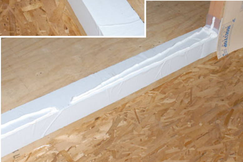
Figure 4. In the barrier method, polyurethane sealant is applied in two continuous \frac{5}{8} -inch-diameter beads all the way across the door pan and 6 inches up both trimmers, one toward the front of the rough opening and one toward the rear (left). In the drainage method, the sealant is applied in elongated triangles, with a 2- to 3-inch gap in the center to allow water to escape (below left). An L-shaped metal dam embedded in sealant and fastened to the floor after the door is installed directs water toward the drainage gap (below right).
