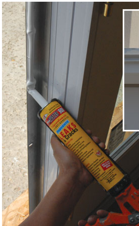
Figure 5. Nailing fins get a continuous bead of sealant before installation (left); the upper corners are protected by a pair of flexible corner flashings bedded in the sealant (above). These flashings also help build out the top of the door to match the base, keeping the unit plumb after installation.
