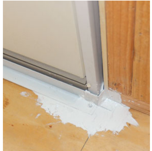
Figure 4. In the barrier method, polyurethane sealant is applied in two continuous \frac{5}{8} -inch-diameter beads all the way across the door pan and 6 inches up both trimmers, one toward the front of the rough opening and one toward the rear (left). In the drainage method, the sealant is applied in elongated triangles, with a 2- to 3-inch gap in the center to allow water to escape (below left). An L-shaped metal dam embedded in sealant and fastened to the floor after the door is installed directs water toward the drainage gap (below right).
