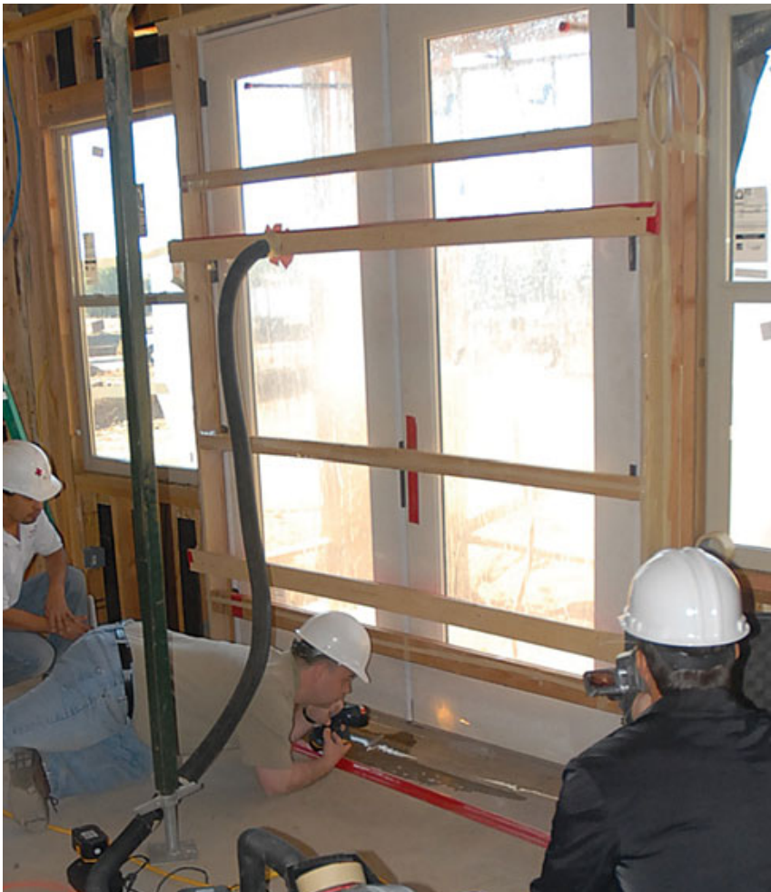
Figure 1. French doors have a reputation as being leak-prone, but most problems stem from improper installation. Here, a spray-rack test shows water leaking between the sill and the subfloor.
