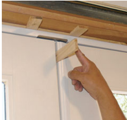
Figure 6. Shims are critical for door performance. They're needed behind every hinge (left) and across the top jamb. Temporarily shimming the gap between the two door sash keeps the unit from distorting or overcompressing the weatherstripping while the door is installed (above).
