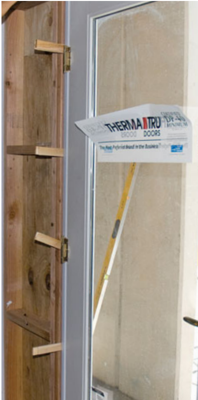
Figure 6. Shims are critical for door performance. They're needed behind every hinge (left) and across the top jamb. Temporarily shimming the gap between the two door sash keeps the unit from distorting or overcompressing the weatherstripping while the door is installed (above).
