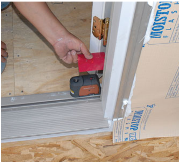
Figure 7. The most accurate way to check if a rough opening or installed door is plumb is with a laser (above), but the easiest way to check for a cross-legged opening or door is with a pair of crisscrossed strings (right). The strings should touch gently in the center.
