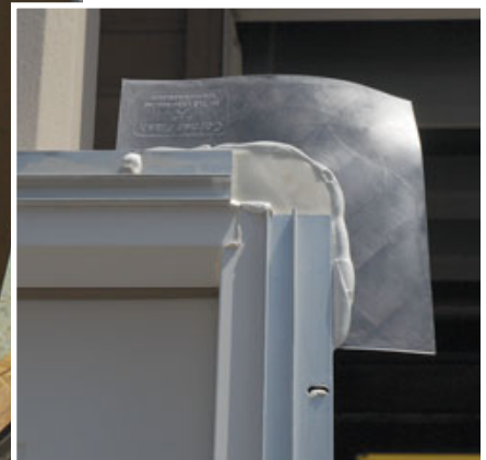
Figure 5. Nailing fins get a continuous bead of sealant before installation (left); the upper corners are protected by a pair of flexible corner flashings bedded in the sealant (above). These flashings also help build out the top of the door to match the base, keeping the unit plumb after installation.
