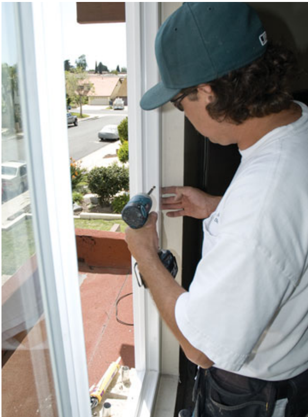
Figure 3. Another fat bead of sealant is applied to the fin before the window is installed (top left). When the diagonals are equal, the window is square in the opening (top right). The window is fastened to the wall framing with 3-inch deck screws driven through the jambs (above); plastic shims prevent the vinyl frames from distorting.
