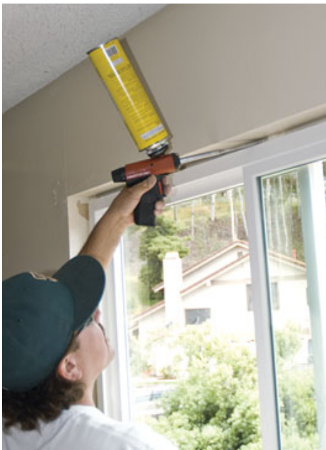
Figure 5. Low-expansion foam sprayed between the frame and the wall air-seals the window (above) and provides backing for self-adhesive vinyl trim tape (above right). A smooth bead of caulk finishes the installation (right).
