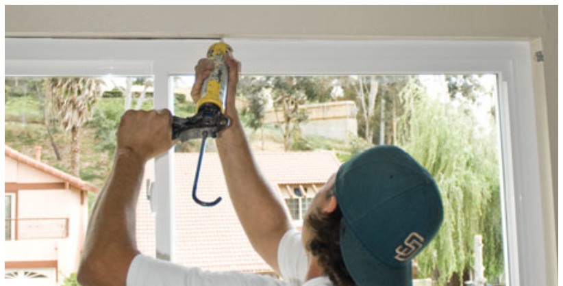
Figure 5. Low-expansion foam sprayed between the frame and the wall air-seals the window (above) and provides backing for self-adhesive vinyl trim tape (above right). A smooth bead of caulk finishes the installation (right).
