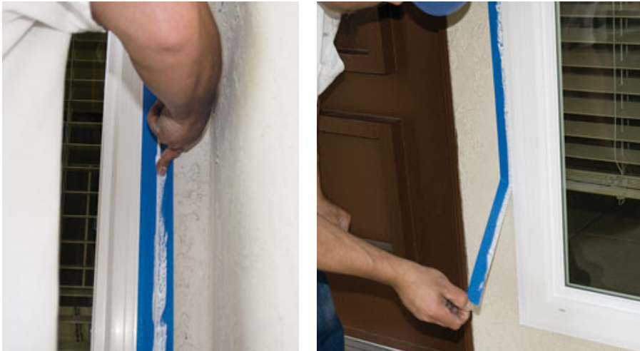
Figure 4. Sealant should be compressed as the window is installed, and tooled after the window is fastened in place, to remove small voids and air bubbles (far left). With a flush window, applying painter's tape to the wall and window fin gives the sealant a straight edge and speeds cleanup (left).
