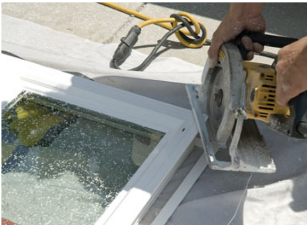
Figure 1. When a finned unit is trimmed to fit a recessed opening, an equal amount should be removed from each fin to ensure that the unit is centered in the opening (top). Vinyl fins can be cut with a utility knife, but a saw is more accurate (center). Rounding off the corners (above) makes it easier to fit the window into the recessed opening.
