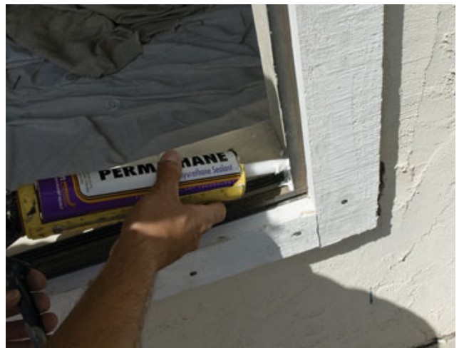
Figure 2. Before the window is installed, the old window frame gets a 1/2-inch-diameter continuous bead of polyurethane sealant (top). Extra sealant pumped into the upper (center) and lower corners (above) prevents water that may have leaked behind the stucco from exiting the wall cavity at the old window frame.
