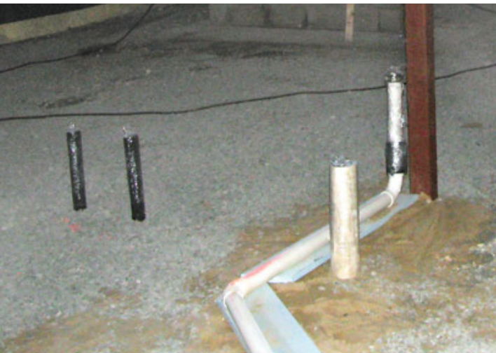
Figure 3. Cured foam sticks tenaciously to most surfaces. Plastic food wrap protects these plumbing stubs from the overspray.
