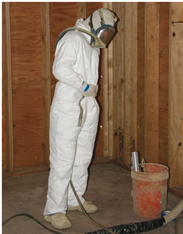
Figure 5. A supplied-air respirator is a must when spraying foam. A layer of clear plastic wrap keeps the face shield clean for repeat use.
