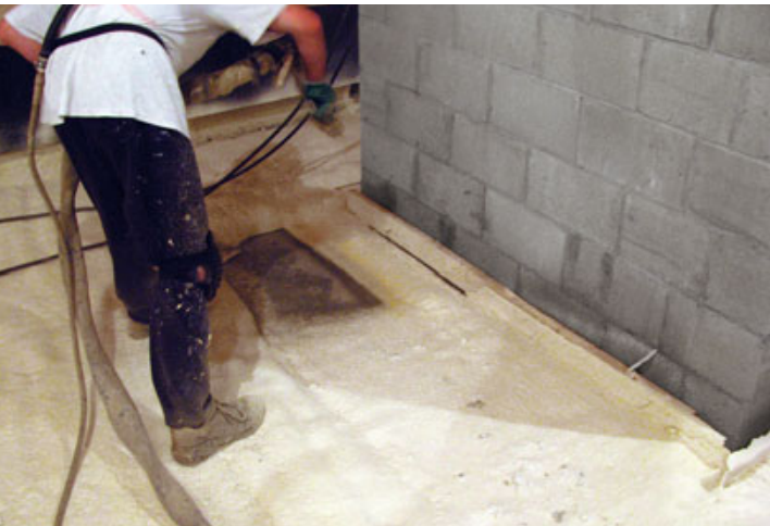
Figure 2. The foam can be walked on only minutes after spraying, permitting multiple layers without significant delay. The 2x4 at this chimney base will be removed after spraying to provide the code-required gap between the flue and the foam.
