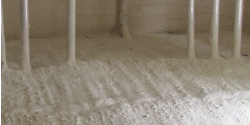
Figure 1. Plumbing penetrations can be tricky to plug with rigid foam board; SPF seals seamlessly around obstacles with a few passes of the spray gun.
