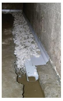
Adding an interior perimeter drain to an existing basement is cheaper and easier than exterior waterproofing. Drains like the one shown here cost in the neighborhood of \$40 per linear foot.
