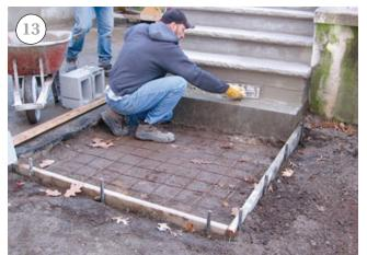
for waste. We used a circular saw and an angle grinder, both equipped with diamond blades, to cut the stone (11). When we set the treads, we pitched them so that water would drain away from the steps.
