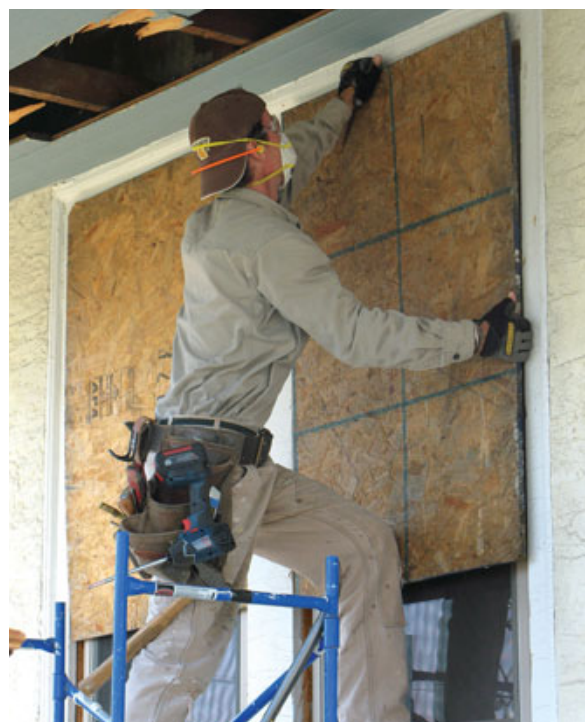
Figure 2. A rolling scaffold helped the author reach the porch ceiling for everything from demo to protecting the windows. Protecting the worksite is part and parcel of renovation work. Include protective materials such as OSB, plus the time to hang it, remove it, and trash it, in your proposal.
