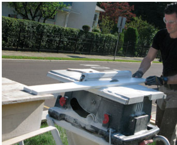
Figure 7. Placing the miter saw and tablesaw close to each other allows the miter saw's table to serve as an outfeed support for the tablesaw.
