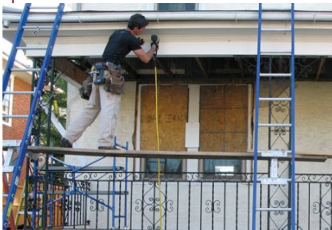
Figure 3. Because porches imply roofs, rehabbing them means you need to work efficiently at a height. Ladder brackets are a great way to support scaffold planks and don't take up a lot of space when you store them.
