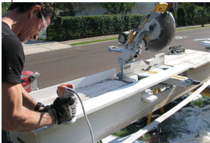
Figure 9. Reproducing an old-house look is fairly easily done on site by using a variety of router bits to shape 1-by stock.
