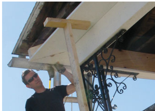
Figure 8. Re-trimming over a gnarly old frame with PVC was easier than using wood. Wood is inevitably slightly cupped or warped; the dead-flat PVC made it easier to wrangle tight miters up in the air. Cleats held by Rockwell Jawhorses made it a one-man job.
