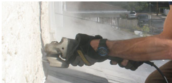
Figure 5. For working on stucco-clad houses, an angle grinder is invaluable. Here, the author cuts in a kerf for flashing. Other uses include cutting around old moldings so they can be removed without damaging the stucco.
