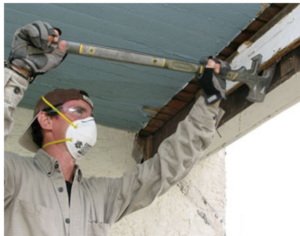
Figure 4. Efficient demolition is as important as efficient construction. Stanley's Fubar III makes quick work of rough tear-out.
