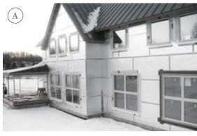
An exterior skin of foil-faced polyiso — with seams taped and windows tightly flashed — helps seal the shell and further reduces thermal bridging (A). Pre-drywall blower-door testing (B) done in conjunction with an infrared camera (C) helped to locate air leaks in the tightly insulated interior (D).
