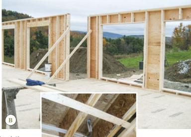
Achieving low heating loads starts with good insulation: Two layers of 2-inch EPS provide a nominal R-26 below the slab (A). Advanced framing techniques like single top plates (B) and two-stud corners (C) reduce thermal bridging.
