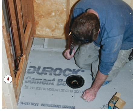
The first thing I did was place the base on the ground and stomp on it. Reassured of its strength, I also tried to peel the membrane away from the plastic structure, but it held firm. Cutting the base to size was easy. The instructions recommend scoring and snapping the base, as you would do with drywall, but with a product this costly I wanted to make sure I had a clean cut. So I cut first from the top, using a utility knife (1), then flipped it over and finished cutting from the back (2).
