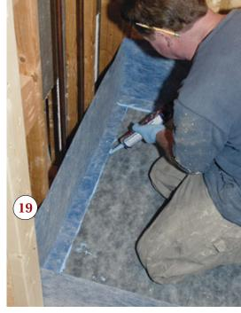
continuous line of squeeze-out (17). After sealing the overlap in the corner (18), I worked back around the perimeter with the caulk gun, laying additional sealant to thoroughly cover the joint between the wall membrane and the base (19).
