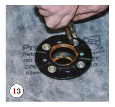
perimeter membrane fabric, leaving enough for about a 4-inch overlap. Then, following the manufacturer's instructions, I prebent a 2-inch leg along one edge (14), which I firmly bedded into a double bead of sealant around the base to create a good bond (15, 16), looking for a
