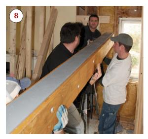
nailed to the walls at each end (8). Then, using a bottle jack, they forced it up into the slot and supported it on temporary wood posts (9). Square hollow-steel posts standing on the slab foundation and welded to the beam provide permanent support (10). New joist hangers completed the installation (11).
