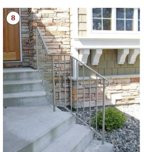
the balusters, nor a 6-inch sphere through the triangular space under the bottom rail.
