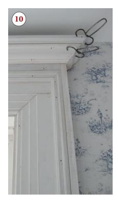
the table saw (9). The backband turns vertically across the head casing for a slightly wider reveal (10).
