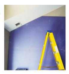
high-density, paper-faced gypsum board; the increased mass and special damping properties of this construction make the drywall effective for high-rated STC wall partitions, says the maker. It costs just under \$2 per square foot.
