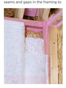
protect against air infiltration, is less toxic than typical expanding foam systems, says the maker. The system costs about \$1 per finished square foot of house more than the company's standard insulation package.
