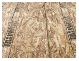
**King-Size Sheets.** *TallWall* lets you sheathe today's taller walls without creating horizontal seams. The extra-long OSB panels come in 9- and 10-foot lengths. When installed vertically, says the maker, the product reduces air infiltration by up to 60 percent and makes the wall assembly much stronger, especially if it overlaps joist areas. A 10-foot panel costs about \$13.50.
