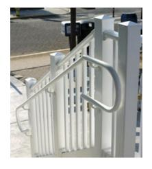
Modified Wood. Titan Wood Limited's *Accoya* pine lumber has been treated with a concentrated form of vinegar in a process called acetylation.
