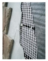
Fiberglass Lath. In contrast to traditional metal lath, woven fiberglass *SpiderLath* is rustproof and unlikely to cut the installer. It's also very light: A 300-square-foot roll weighs 23 pounds. Foam strips running the length of the product provide separation from the substrate and form a seal around nail penetrations. A 4-foot-tall 300-square-foot roll costs \$160.
