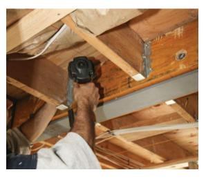
calculate the resulting composite section using a modular ratio to convert a wood section to an equivalent steel section (or vice versa). The modular ratio is the relationship between the elastic moduli of both materials and has a nondimensional value on the order of 14.5 for steel over wood. In other words, steel is about 14.5 times stronger than wood.
