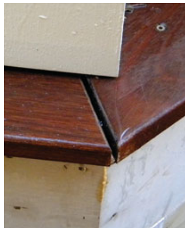
Figure 2. Leaving a gap in a miter joint and routing a radius on the cut ends disguises joint movement.
