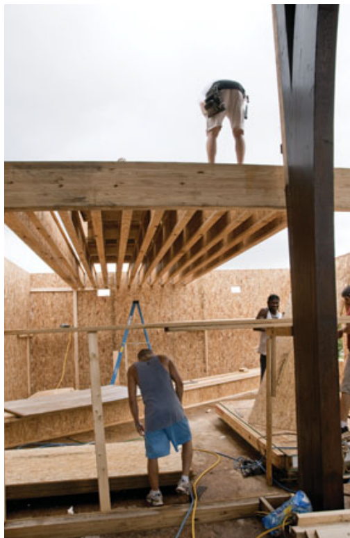
Figure 7. The second-story floor system in the transept addition (above right) hangs between the top of the first-floor wall panels and 6x16 glulam beams that span the openings between the arches of the old structure (above). The 32-foot-long structural ridge beam fit into reinforced pockets in the gable SIPs (right).
