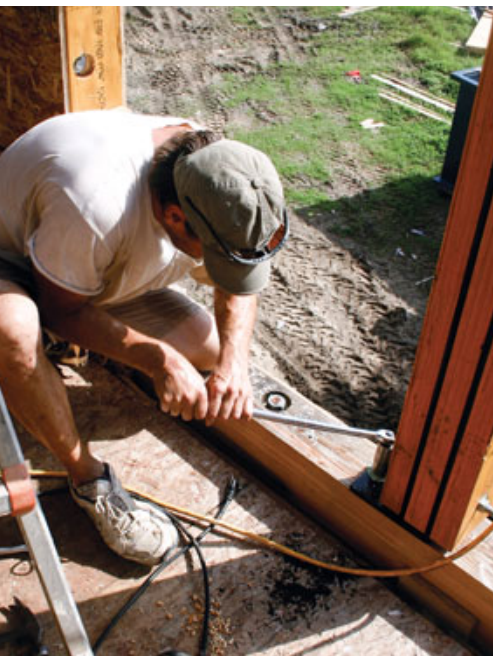
Figure 5. To prevent wind deflection, the tall window walls were reinforced with full-length flitch-beam stiffeners (right), which were bolted to the glulam rim joists (above) and recessed into the wall panels.
