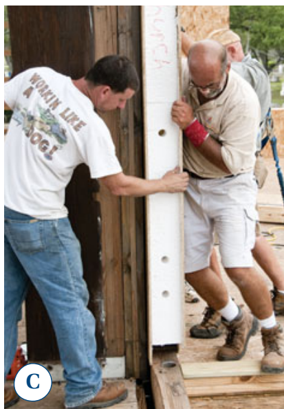
Figure 4. The floor was 14 feet above grade, so man lifts were essential for safe handling of the large panels (A, B). Panel edges were relieved at the bottom to fit over the glulam rim joist, and at the sides and top for the 2-by connecting splines (C). The wall panels were first glued and nailed to the glulam band and splines, then fastened to each other and to existing framing with structural screws (D).
