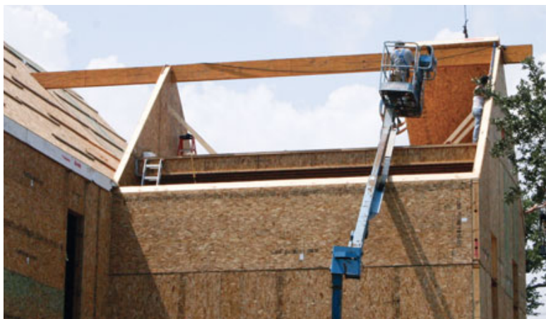
Figure 7. The second-story floor system in the transept addition (above right) hangs between the top of the first-floor wall panels and 6x16 glulam beams that span the openings between the arches of the old structure (above). The 32-foot-long structural ridge beam fit into reinforced pockets in the gable SIPs (right).
