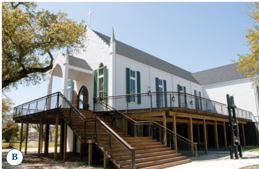
Figure 8. The nonstructural skirt wall (A) and lowered entry deck (B) make the church appear lower to the ground than it actually is, but there’s also elevator access from the finished slab underneath the building (C). With the arches and finish ceiling intact — and the original stained-glass window back in place — the interior looks almost unchanged (D).
