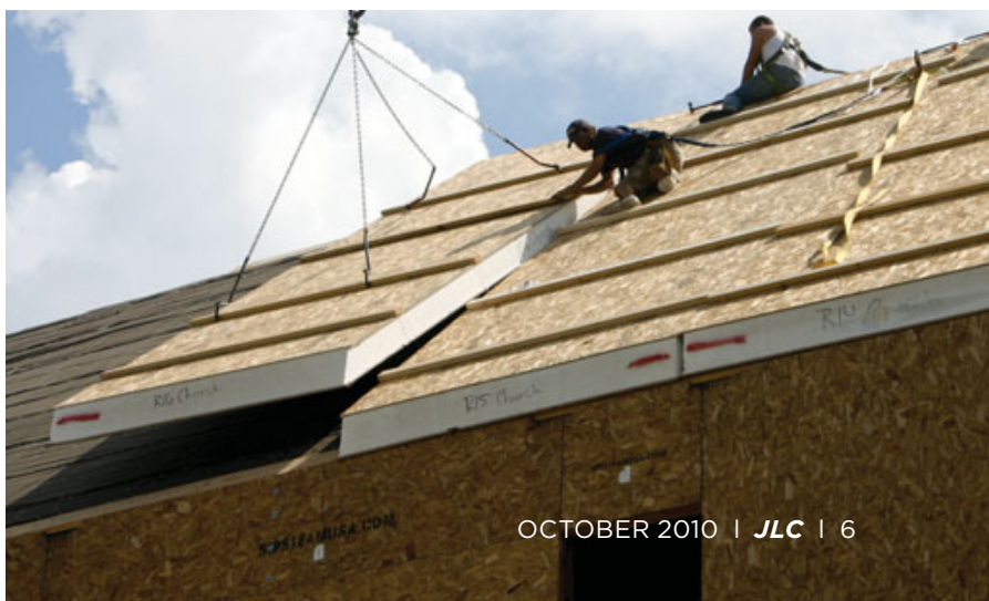
Figure 6. Preinstalled 2-by walk boards reinforced the connection between the lifting hooks and the OSB skins of the roof panels (above, above right). Placing the hooks slightly off-center eliminated camber in the panel, making it easier to slide the edge over the spline of the previous panel (right).
