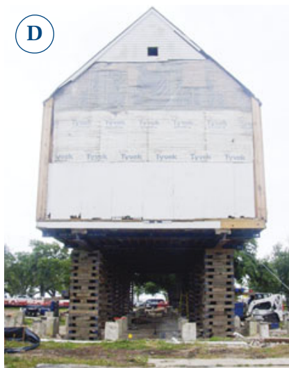
Figure 1. The shoring crew first disconnected the floor framing from the foundation by cutting the steel bolts embedded in the short concrete piers (A), then installed cribbing and hydraulic jacks for lifting the building (B). Each jack was connected to a hydraulic manifold powered by a diesel engine (C), which was able to lift the 3,000-square-foot structure more than 10 feet with less than \frac{3}{8} -inch difference in elevation between any of the 10 lifting points (D).
