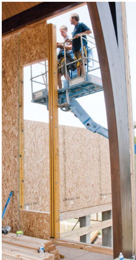
Figure 5. To prevent wind deflection, the tall window walls were reinforced with full-length flitch-beam stiffeners (right), which were bolted to the glulam rim joists (above) and recessed into the wall panels.
