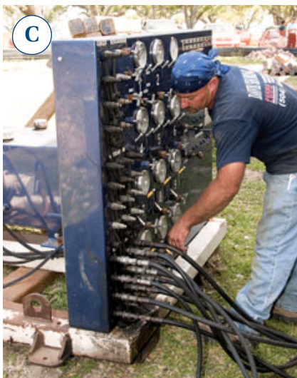
Figure 1. The shoring crew first disconnected the floor framing from the foundation by cutting the steel bolts embedded in the short concrete piers (A), then installed cribbing and hydraulic jacks for lifting the building (B). Each jack was connected to a hydraulic manifold powered by a diesel engine (C), which was able to lift the 3,000-square-foot structure more than 10 feet with less than \frac{3}{8} -inch difference in elevation between any of the 10 lifting points (D).
