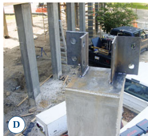
Figure 2. The rebar for new grade beams and pier extensions was epoxied to the original piers (A). Formwork for the pier extensions stopped a foot shy of the raised building to allow for setting the anchor bolt-studded cap plates and pumping the concrete (B). Diagonal steel rods provide lateral bracing for the exposed portions of the piers (C); note the cold joint at the base of each pier between the old pier and the pier extensions. Steel brackets welded to the cap plates anchor the transept framing to the foundation (D).
