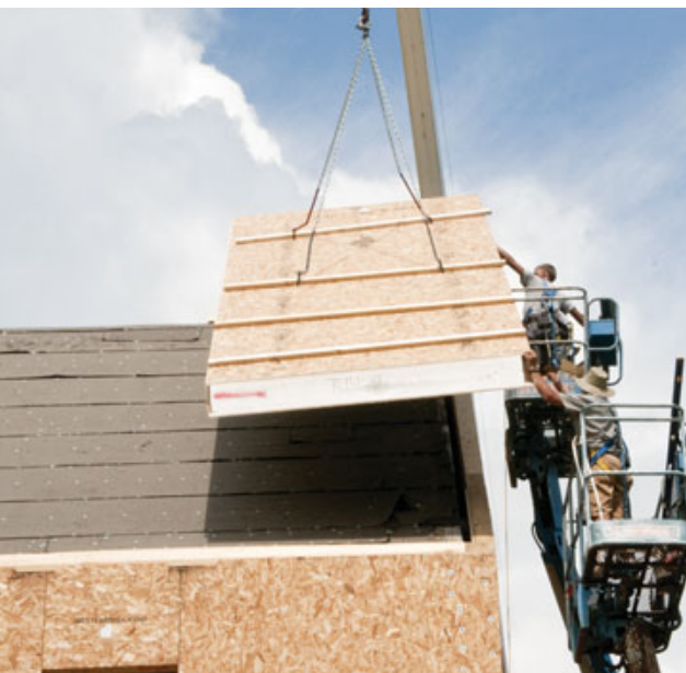
Figure 6. Preinstalled 2-by walk boards reinforced the connection between the lifting hooks and the OSB skins of the roof panels (above, above right). Placing the hooks slightly off-center eliminated camber in the panel, making it easier to slide the edge over the spline of the previous panel (right).
