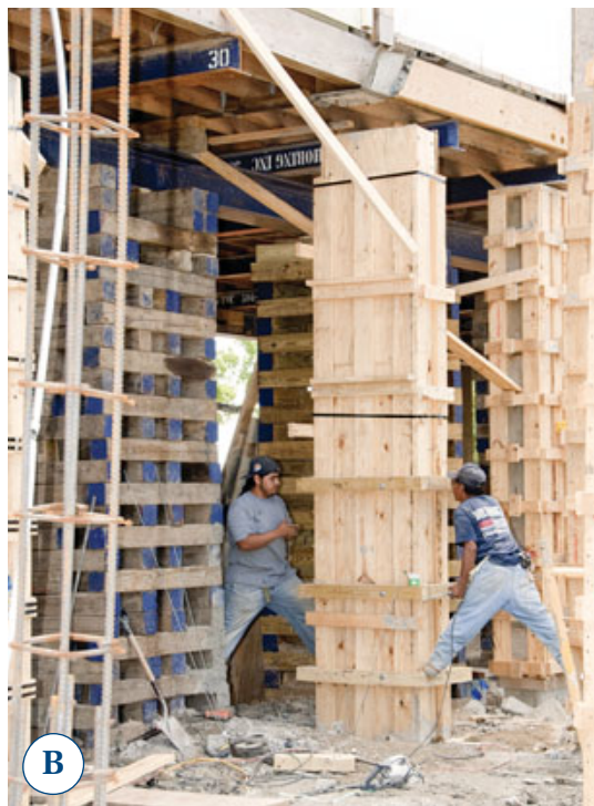
Figure 2. The rebar for new grade beams and pier extensions was epoxied to the original piers (A). Formwork for the pier extensions stopped a foot shy of the raised building to allow for setting the anchor bolt-studded cap plates and pumping the concrete (B). Diagonal steel rods provide lateral bracing for the exposed portions of the piers (C); note the cold joint at the base of each pier between the old pier and the pier extensions. Steel brackets welded to the cap plates anchor the transept framing to the foundation (D).
