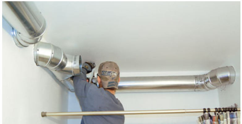
Figure 7. If the duct can't be placed in the wall, another possibility is to route it through a concealed area, such as a closet (above left). When all else fails, it can be installed in the room (above) and boxed in later on (left).
