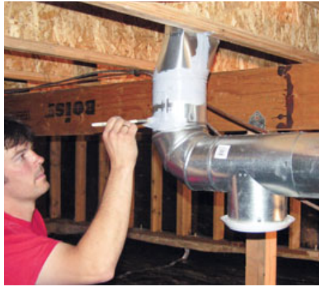
Figure 8. Joints in metal duct must be sealed with mastic (left) or butyl tape (right). Here, a joist is obstructing the back of the duct riser, so the tape is positioned all the way around before the release paper is peeled off and the tape pressed in place.
