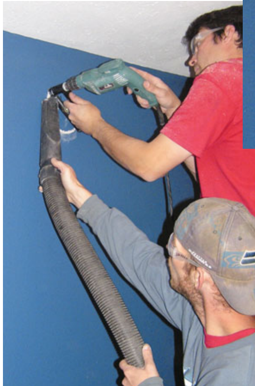
Figure 6. As a drill-operated hole saw cuts through the finished drywall, a shop vac collects dust before it has a chance to spread (left). The oval riser behind the drywall was previously cut out to accept the wall register (above), which can now simply be snapped in place.
