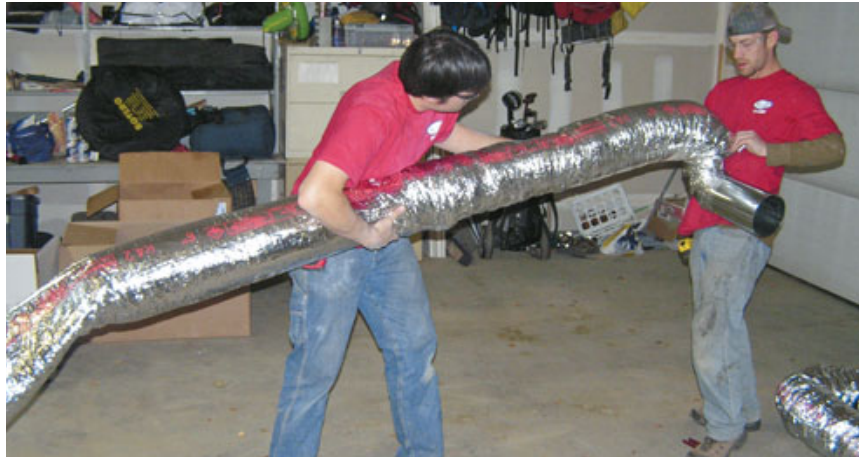
Figure 2. Where a cold-side run of rigid duct is unavoidable, as in a garage, the pre-assembled duct can be slipped inside the foil-faced insulating jacket from a length of flex duct.
