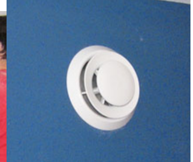
Figure 6. As a drill-operated hole saw cuts through the finished drywall, a shop vac collects dust before it has a chance to spread (left). The oval riser behind the drywall was previously cut out to accept the wall register (above), which can now simply be snapped in place.
