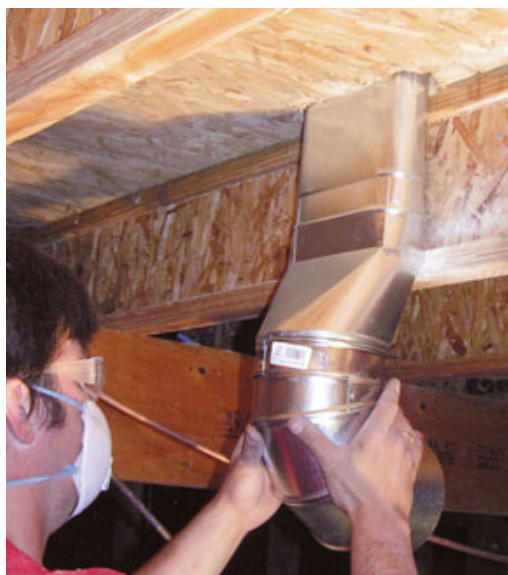
Figure 5. After one end of an oval riser is capped and sealed with tape (above left), it's slipped into a hole cut through the subfloor and bottom plate of a partition wall (above). A round hole in cut in the side of the riser (not visible here) will later accept a wall register. The lower end of the riser transitions to a 6-inch round duct for connection to the warm-side run leading to the HRV (left).
