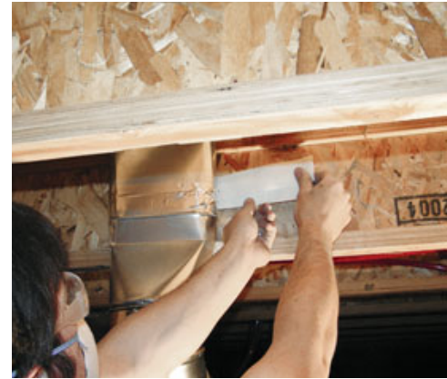
Figure 8. Joints in metal duct must be sealed with mastic (left) or butyl tape (right). Here, a joist is obstructing the back of the duct riser, so the tape is positioned all the way around before the release paper is peeled off and the tape pressed in place.
