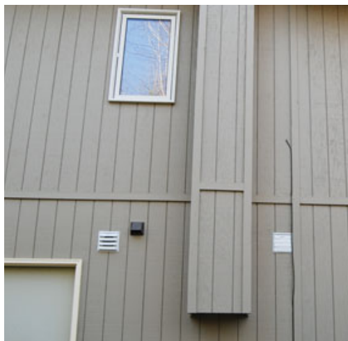
Figure 3. A duct carrying stale air from the HRV passes through the rim joist and connects to a riser hood (above left) that directs the exhaust to an exit point 18 inches above grade (above). In the installation shown at left, the exhaust and intake are high in the wall and separated 6 feet horizontally to meet code. The intake louvers are permanently open, but the exhaust louvers open only when the HRV is running.
