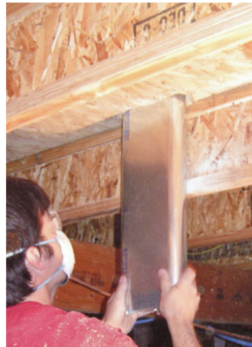
Figure 5. After one end of an oval riser is capped and sealed with tape (above left), it's slipped into a hole cut through the subfloor and bottom plate of a partition wall (above). A round hole in cut in the side of the riser (not visible here) will later accept a wall register. The lower end of the riser transitions to a 6-inch round duct for connection to the warm-side run leading to the HRV (left).
