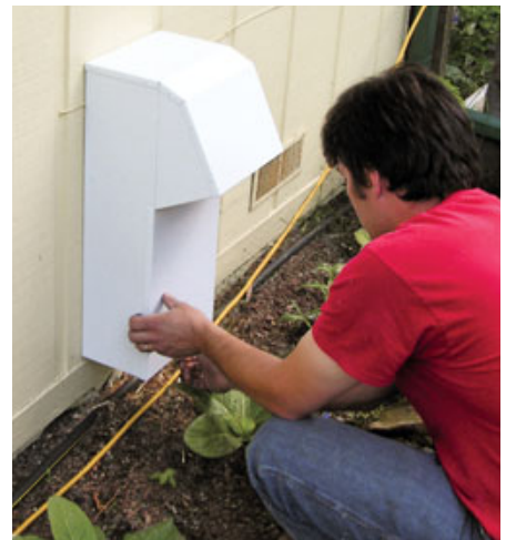
Figure 3. A duct carrying stale air from the HRV passes through the rim joist and connects to a riser hood (above left) that directs the exhaust to an exit point 18 inches above grade (above). In the installation shown at left, the exhaust and intake are high in the wall and separated 6 feet horizontally to meet code. The intake louvers are permanently open, but the exhaust louvers open only when the HRV is running.
