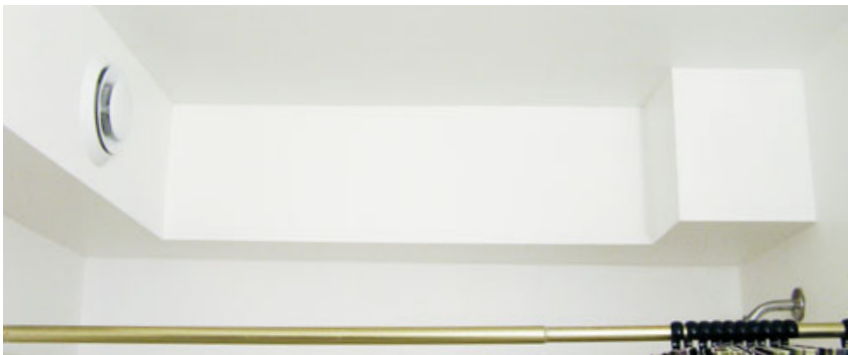
Figure 7. If the duct can't be placed in the wall, another possibility is to route it through a concealed area, such as a closet (above left). When all else fails, it can be installed in the room (above) and boxed in later on (left).
