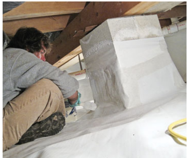
Figure 3. After removing any loose tape (left), the authors applied mesh tape and mastic to every lap and cut around the piers (below). To make sure they sealed every joint, they worked the piers as a team, positioning themselves on each side; this also reduced unnecessary movement on the membrane as the mastic set up.
