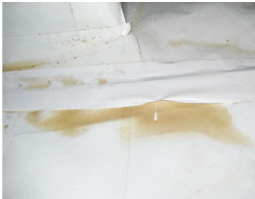
Figure 1. In spite of being taped, many of the joints in the CleanSpace liner were leaking liquid water, as evidenced by the dirt stains left behind.
