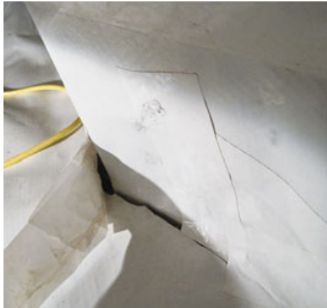
Figure 3. After removing any loose tape (left), the authors applied mesh tape and mastic to every lap and cut around the piers (below). To make sure they sealed every joint, they worked the piers as a team, positioning themselves on each side; this also reduced unnecessary movement on the membrane as the mastic set up.
