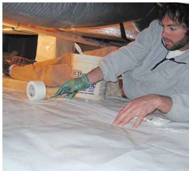
Figure 1. In spite of being taped, many of the joints in the CleanSpace liner were leaking liquid water, as evidenced by the dirt stains left behind.
