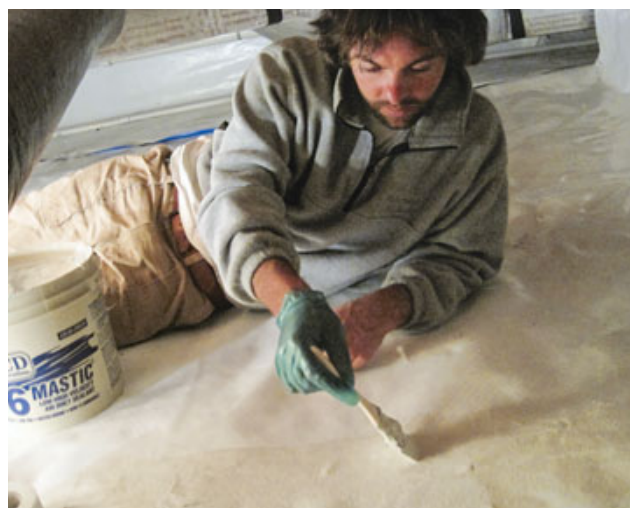
Figure 2. Fiberglass mesh tape (top) followed by a thick coating of duct mastic created rugged, waterproof seams. The self-sticking mesh tape held the overlapping plastic sheets in place as the mastic set up.
