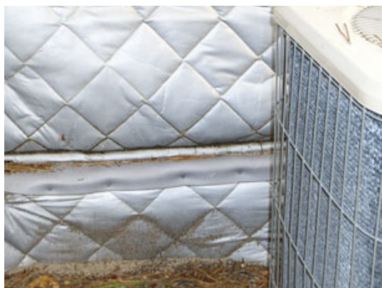
Figure 1. A simple barrier lined with acoustic blankets will absorb and block most of the noise produced by this AC condenser. The blankets consist of a UV-protected composite 1-pound mass-loaded vinyl barrier faced with a 2-inch-thick quilted fiberglass absorber. Note how the blanket extends below grade (left).
