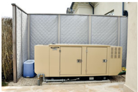
Figure 2. This 10-foot-tall barrier will provide almost twice the noise reduction of a 5-foot-tall barrier, even with clearances between the generator and enclosure limited because of the existing landscape design and zoning constraints.
