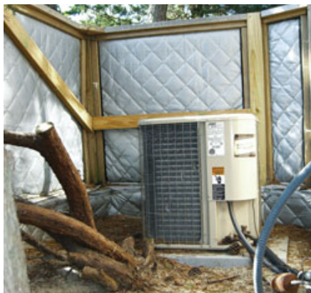
Figure 1. A simple barrier lined with acoustic blankets will absorb and block most of the noise produced by this AC condenser. The blankets consist of a UV-protected composite 1-pound mass-loaded vinyl barrier faced with a 2-inch-thick quilted fiberglass absorber. Note how the blanket extends below grade (left).
