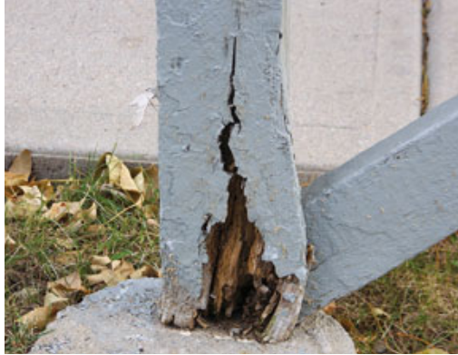
Figure 5. Lateral forces applied to the deck are transmitted through the cross bracing attached to the base of the support post. A combination of decay and lateral forces has begun to rip apart this post.
