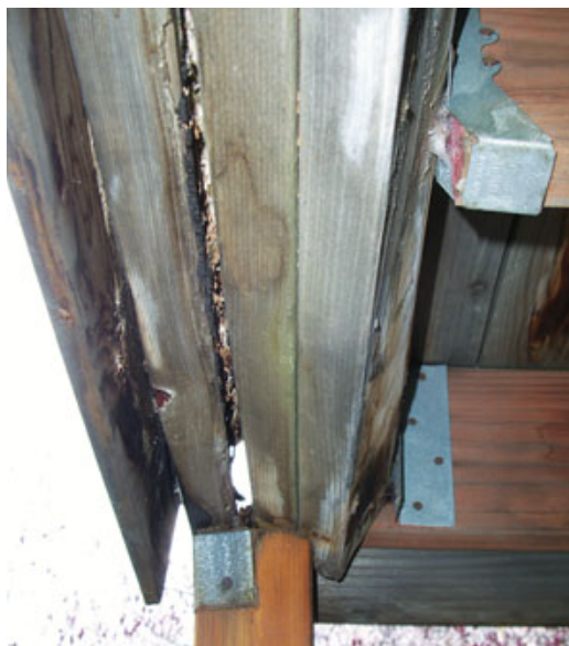
Figure 4. Moisture trapped between its members has rotted this beam, which is at risk for imminent collapse.
