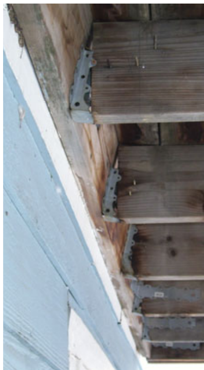
Figure 3. The rotating ledger in this photo was a complete surprise to the homeowner. This ledger has completely pushed the joists out of the hangers, and the deck is at risk of collapse. Ledgers that slowly pull away often rotate from the top, making the hazard less noticeable from beneath.
