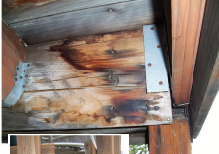
Figure 1. From a garden-level window under the deck, this beam looks merely water-stained (above). The fascia and the guard balusters were in good shape and were even recently stained. The owner thought the deck was fine, but with a slight tug at the fascia, the beam fell apart (left). Though the redwood fascia and decking were able to resist rot, the fir framing had deteriorated from trapped moisture.
