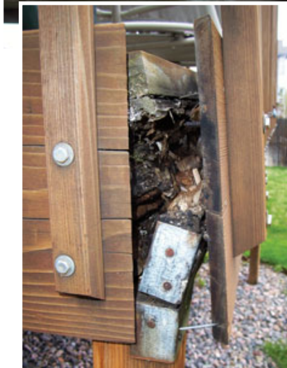
Figure 1. From a garden-level window under the deck, this beam looks merely water-stained (above). The fascia and the guard balusters were in good shape and were even recently stained. The owner thought the deck was fine, but with a slight tug at the fascia, the beam fell apart (left). Though the redwood fascia and decking were able to resist rot, the fir framing had deteriorated from trapped moisture.
