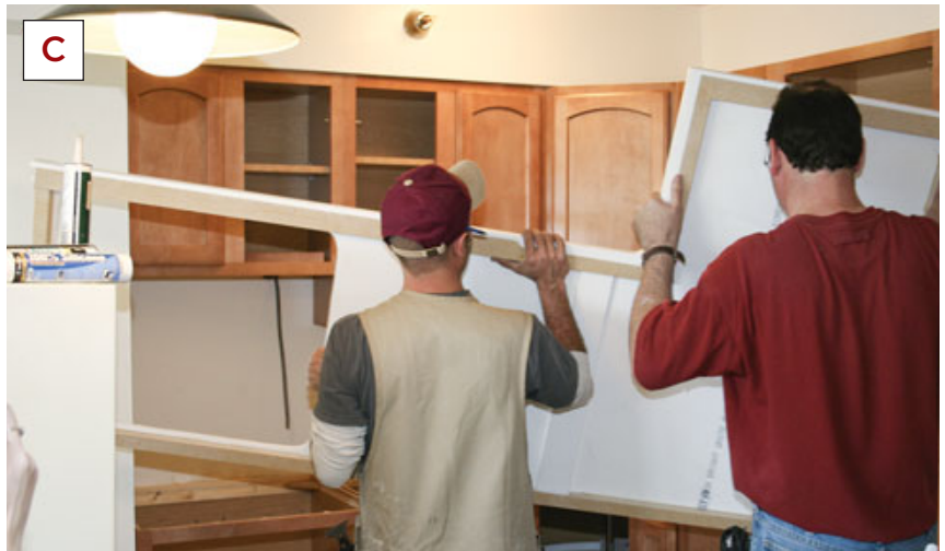
Figure 6. To contain dust, sink cutouts were made in the field office (A); then the Staron solid-surface countertops were wheeled to the apartment on a drywall cart and installed (B,C). By the end of the job, the author's three-man crew was remodeling six kitchens per week (D).
