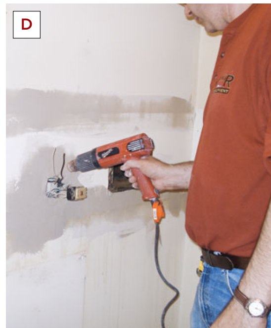
Figure 4. Although each kitchen took only about an hour to demo (A), some needed minor stop-valve relocation (B) and all needed new switched undercabinet lighting, which required careful coordination with plumbing and electrical subs to keep the job on schedule. Patching holes and repainting walls was the most time-consuming part of the job (C), but warming up the setting compound with a heat gun helped speed up the process (D).
