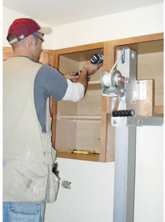
Figure 5. While one crew member patched and painted, another preassembled upper cabinets in the hallway (above left). A cabinet lift made it easy to wheel the assembled cabinets into the apartment and lift them into place (above). Base units were installed after the upper cabinets were in place (left).
