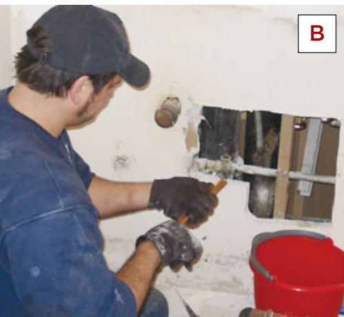
Figure 4. Although each kitchen took only about an hour to demo (A), some needed minor stop-valve relocation (B) and all needed new switched undercabinet lighting, which required careful coordination with plumbing and electrical subs to keep the job on schedule. Patching holes and repainting walls was the most time-consuming part of the job (C), but warming up the setting compound with a heat gun helped speed up the process (D).
