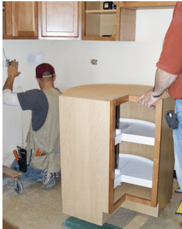
Figure 5. While one crew member patched and painted, another preassembled upper cabinets in the hallway (above left). A cabinet lift made it easy to wheel the assembled cabinets into the apartment and lift them into place (above). Base units were installed after the upper cabinets were in place (left).
