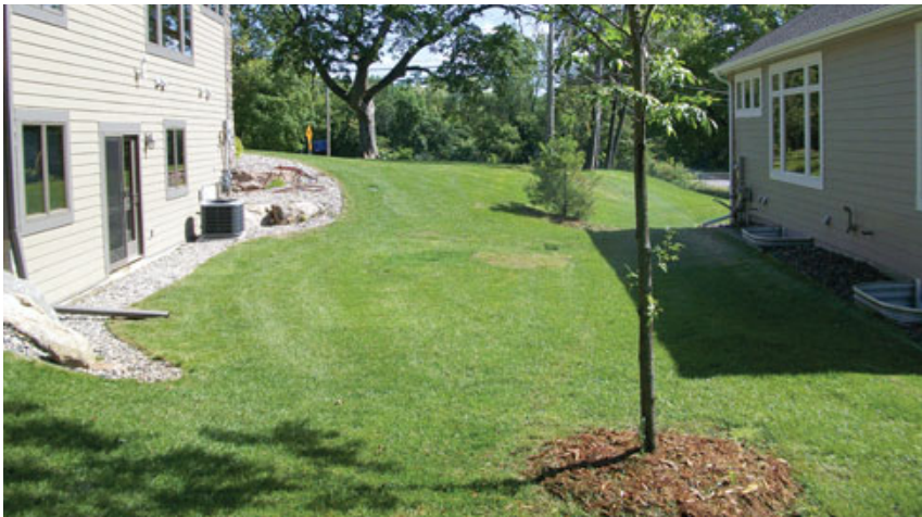
Figure 1. The existing grade channeled runoff between the small evergreen at the center of this photo (taken facing the road) and the corner of the dwelling at right. Digging a swale to divert runoff to the street — as specified by the original plan — would have required tearing up existing landscaping and, most likely, removing the mature tree at the rear of the photo.
