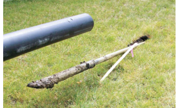
Figure 3. The controls on the horizontal boring rig allow the operator (left) to “steer” the bit left, right, up, or down. On this job, the angled bit emerged from the soil almost exactly on target (above) — note the toppled marker stake leaning against the boring shaft.
