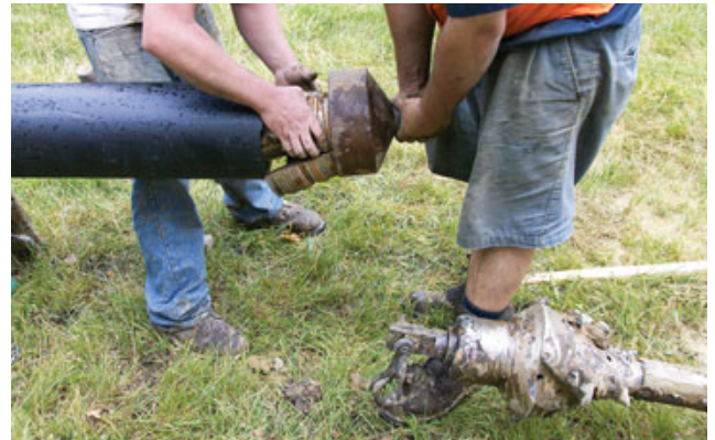
Figure 6. After the boring bit is replaced with the back-reaming bit (above left), which will smooth and enlarge the hole, a sleeved pipe puller is secured to the pipe's downhill end; it grips the pipe like an enormous expansion bolt (above). Then the pipe puller and bit are joined by a swiveling shackle (left) that allows the bit to spin without transmitting that rotation to the pipe, and the operator backs the bit back through the borehole, drawing the pipe in after it.
