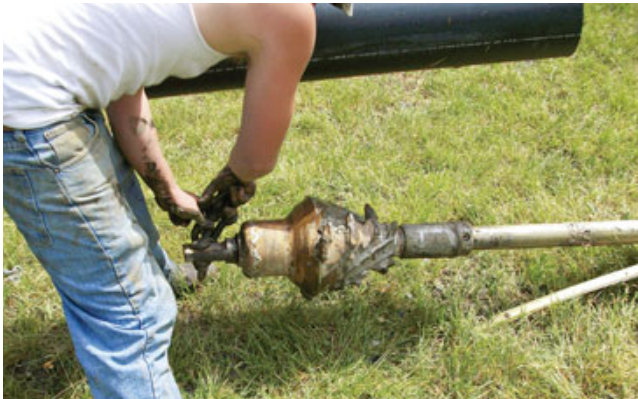
Figure 5. While no one would mistake the welded full-length pipe for a length of garden hose, it does have enough flexibility to conform to irregularities in the borehole.
