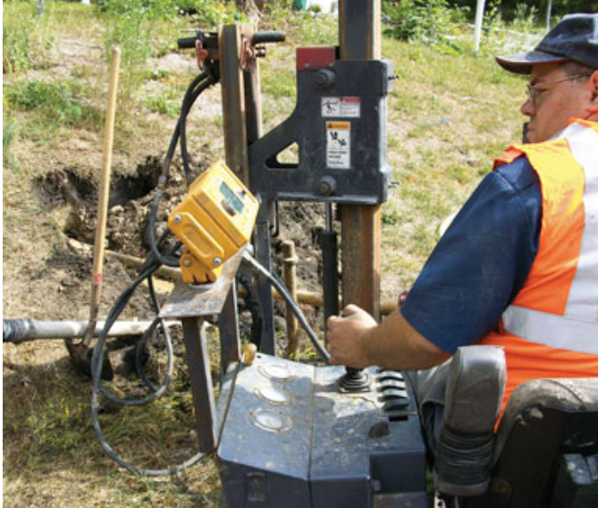
Figure 3. The controls on the horizontal boring rig allow the operator (left) to “steer” the bit left, right, up, or down. On this job, the angled bit emerged from the soil almost exactly on target (above) — note the toppled marker stake leaning against the boring shaft.
