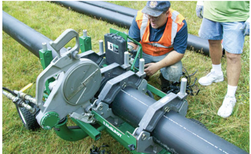
Figure 4. Once two lengths of pipe have been clamped to the pipe-fusing machine, the rotary cutter head precisely squares the ends. The area of the butt joint is then brought up to temperature with an on-board electric heating unit, and the softened ends are forced together with a hydraulic ram.
