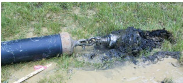
Figure 6. After the boring bit is replaced with the back-reaming bit (above left), which will smooth and enlarge the hole, a sleeved pipe puller is secured to the pipe's downhill end; it grips the pipe like an enormous expansion bolt (above). Then the pipe puller and bit are joined by a swiveling shackle (left) that allows the bit to spin without transmitting that rotation to the pipe, and the operator backs the bit back through the borehole, drawing the pipe in after it.
