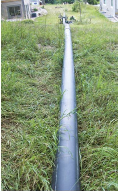
Figure 5. While no one would mistake the welded full-length pipe for a length of garden hose, it does have enough flexibility to conform to irregularities in the borehole.
