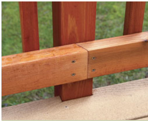
Figure 2. The guardrail posts anchor to the outside of the rim joists, so only one course of decking had to be notched at the rims. Installing the decking from the rim toward the house placed a full-width board above the rim for easy notching and attachment.
