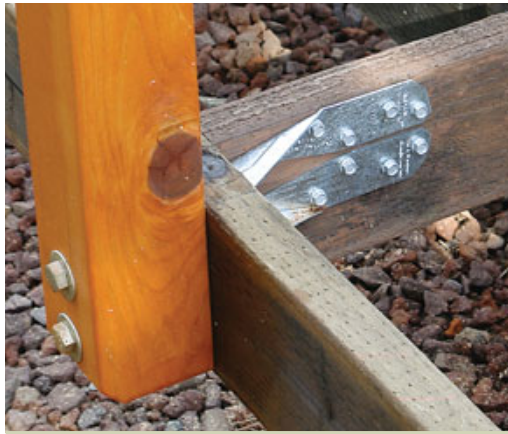
Figure 1. Simpson Strong-Tie's DTT2Z connectors anchor the guardrail posts to 2x6 joists, but deeper joists would have made the guardrails even stronger.
