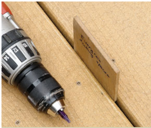
Figure 3. EverGrain deck boards must be spaced at least ⅛ inch apart from side to side, but this larger, 7/32-inch gap is less likely to clog with debris. GRK's star bit drove more than 1,000 Kameleon composite-deck screws with no cam-out.
