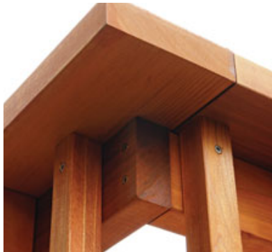
Figure 6. Unlike single corner posts, double corner posts make it easy to butt rather than miter your guardrail caps at the corners. Miter joints can look great at first, but butt joints can look clean and sturdy and tend to age more gracefully than miters do.
