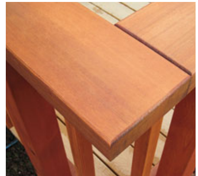
Figure 6. Unlike single corner posts, double corner posts make it easy to butt rather than miter your guardrail caps at the corners. Miter joints can look great at first, but butt joints can look clean and sturdy and tend to age more gracefully than miters do.
