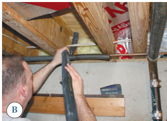
Figure 5. The Velux solar collectors were simply screwed directly to the roof sheathing (A). After running the fluid lines to the utility room (B), the installers made connections at the manifold assembly, which includes a pump, gauges, and controls (C). A pressure tank and insulated storage tank complete the installation (D).
