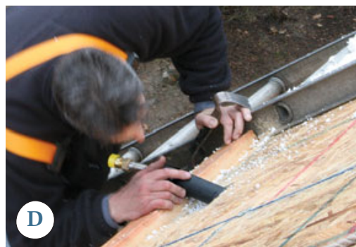
Figure 4. The solar installer uses a recip saw to cut one of the penetrations needed for the fluid pipe loop between the collectors and the utility room (A). Inside, a worker makes a hole in the ceiling several feet away, then scoops out a recess with a hot knife (B). Working from this access point, a worker uses a long drill bit to locate the penetration and create a tunnel to pull the pipe through (C). Snaking the pipes through the panels to the basement proved to be tricky (D).
