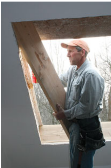
Figure 2. After the opening is made, the crew uses a "hot knife" (far left) to create a recess for 2x10 framing around the edges (left). Above, the finished skylight well.
