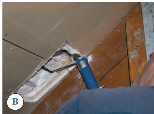
Figure 4. The solar installer uses a recip saw to cut one of the penetrations needed for the fluid pipe loop between the collectors and the utility room (A). Inside, a worker makes a hole in the ceiling several feet away, then scoops out a recess with a hot knife (B). Working from this access point, a worker uses a long drill bit to locate the penetration and create a tunnel to pull the pipe through (C). Snaking the pipes through the panels to the basement proved to be tricky (D).
