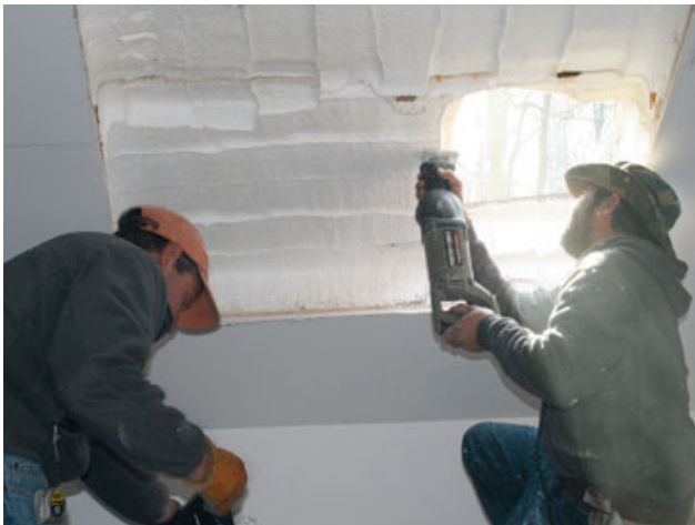
Figure 1. After laying out the skylights from the interior and removing the drywall (top), the installer transfers the location to the roof (center). The bulk of the foam is removed with a recip saw (above).
