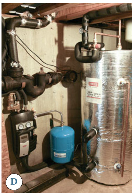
Figure 5. The Velux solar collectors were simply screwed directly to the roof sheathing (A). After running the fluid lines to the utility room (B), the installers made connections at the manifold assembly, which includes a pump, gauges, and controls (C). A pressure tank and insulated storage tank complete the installation (D).
