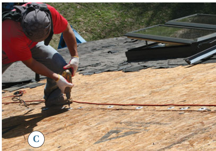
Figure 3. A vertical ripple in the shingles (A) was caused by a slight displacement in the roof panels' edges (B). To make sure the surface was flat before reshingling, the author secured the edges of the panels with washer screws driven into the framing (C), then added another layer of OSB sheathing over the entire roof (D).
