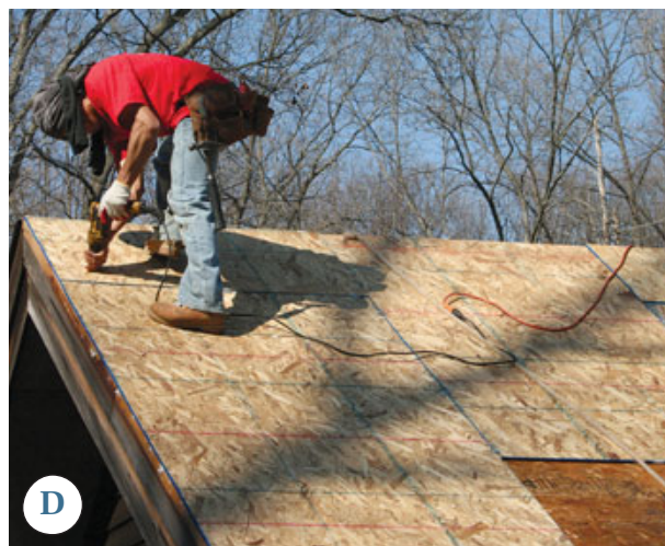
Figure 3. A vertical ripple in the shingles (A) was caused by a slight displacement in the roof panels' edges (B). To make sure the surface was flat before reshingling, the author secured the edges of the panels with washer screws driven into the framing (C), then added another layer of OSB sheathing over the entire roof (D).
