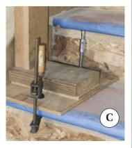
The jig is held in place at the back with a simple expandable compression clamp made from two 5/8-inch-diameter bolts joined by a threaded rod coupler; a quick-release bar clamp holds down the front. I use the same technique to secure my rail jack (C).
